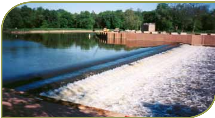
Figure 7. Island Farm Weir stepped spillway modification.
