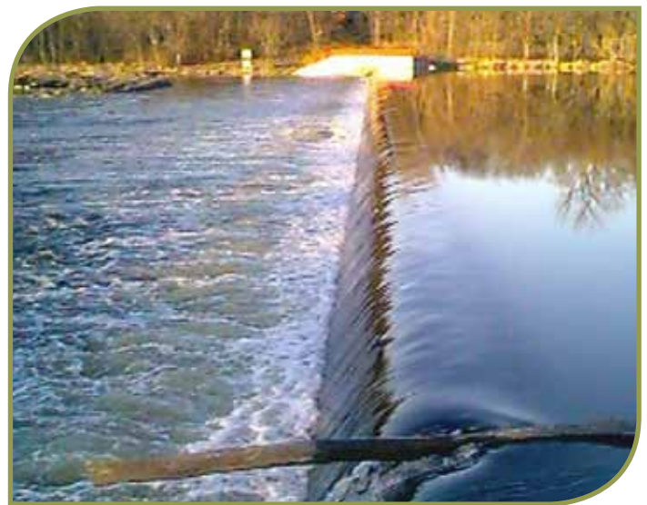
Figure 8. Yorkville Dam on the Fox River.
