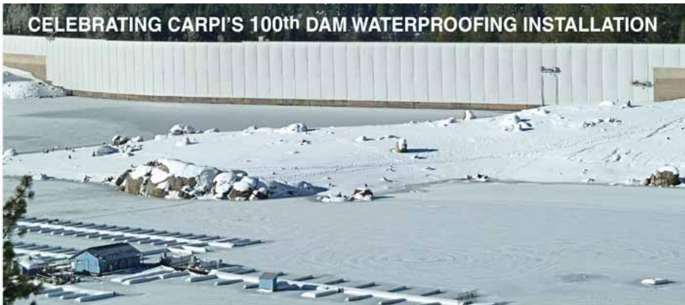
**SHAVER LAKE DAM - USA - January 2011 - (Phase 1 of 2) Waterproofing of a concrete gravity dam with exposed PVC geomembrane**
