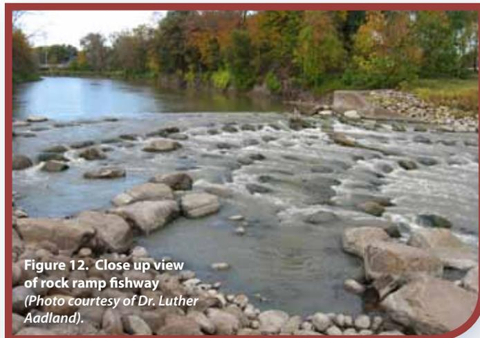
**Figure 12. Close up view of rock ramp fishway (Photo courtesy of Dr. Luther Aadland).**
