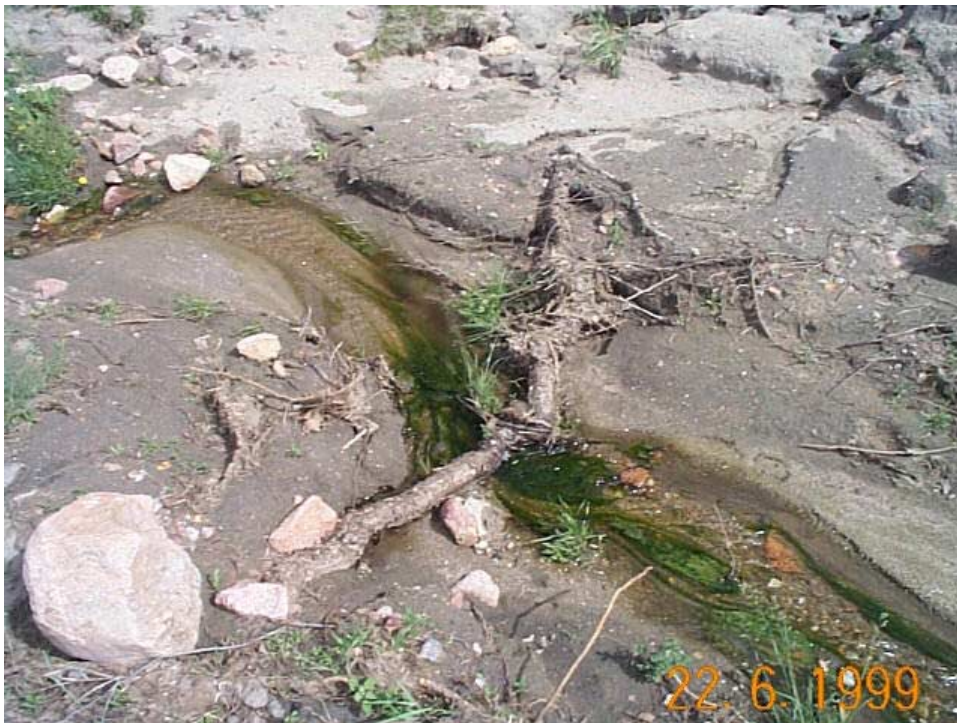
Figure 3. Large pine root located in the channel of the breach opening of a failed Air Force Academy waste lagoon pond dam (David Eyre, Senior Civil Engineer, Air Force Academy, Colorado, 1999).
