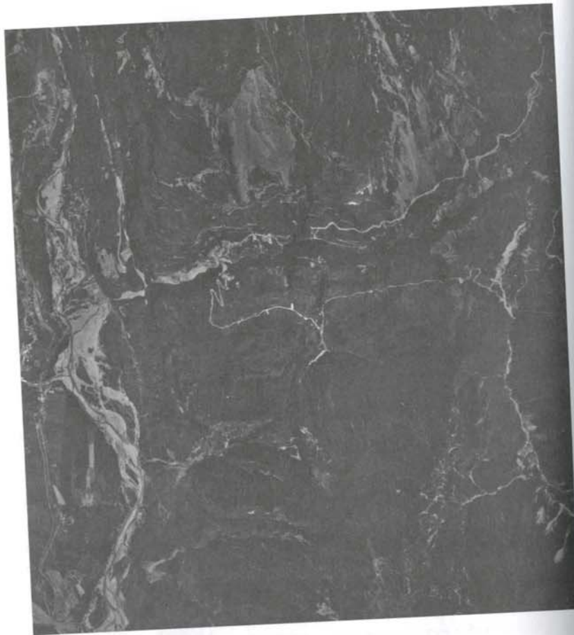
Figure 7-5. Aerial photograph of site before slide. Source: Hendron and Patton (1985).
