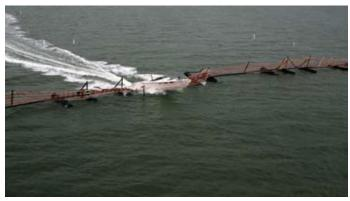
Figure 3: Net Boat Barrier Source: Existing Barrier and Less Than Lethal Technologies, University of Kentucky, March 2012.
