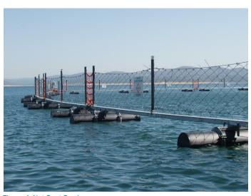
Figure 4: Net Boat Barrier Source: Bureau of Reclamation
