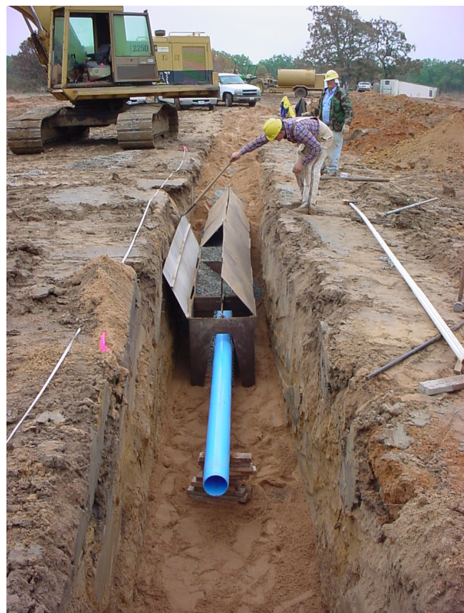
Figure 26A-3 Double filter surrounding collector pipe
