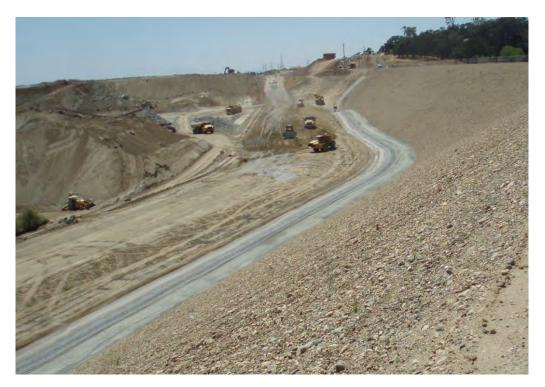
Figure G14. Two-stage filter being installed within overlay at MIAD in California. The filter is the light gray band crossing the picture from the lower left corner.
