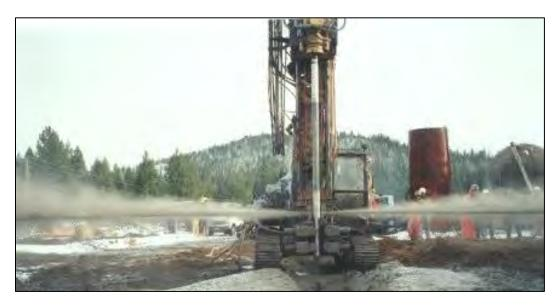
Figure G11. Jet-grout blocks in the foundation of Wickiup Dam.
