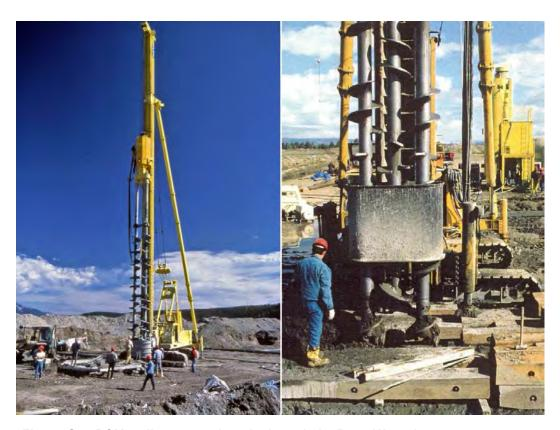
Figure G4. DSM wall construction, Jackson Lake Dam, Wyoming.
