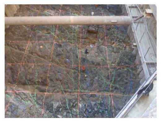
Figure G15. Bedrock painted for geologic mapping and photogrammetry at the bottom of the MIAD key block (2011).
