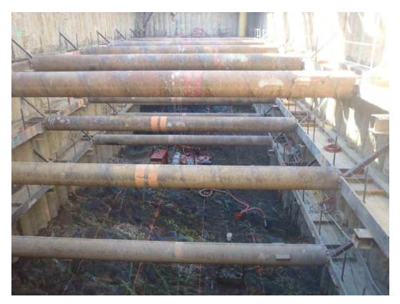
Figure G4b. Excavation bracing for the key block at MIAD, Folsom, California (2011).
