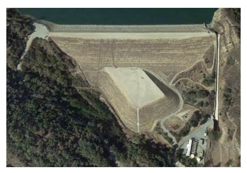
Figure G17a. Casitas Dam stability berm and widened crest.
