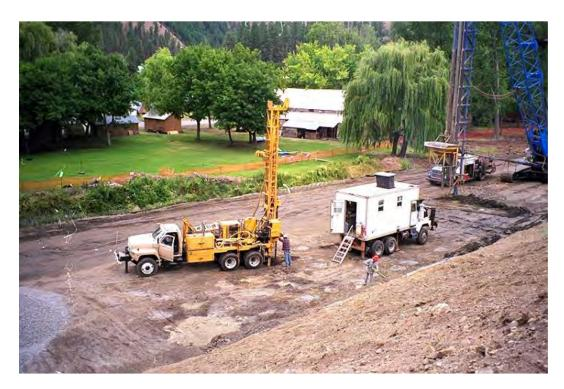
Figure G2. Verification testing with SPT and CPT to confirm sufficient densification by Stone Column Construction at Salmon Lake Dam. Stone column equipment appears at the far right side of the photograph.
