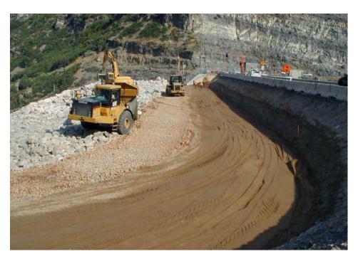
Figure G18. Placement of flowthrough rockfill, transition, and filter zones, downstream to upstream (left to right), Pineview Dam modification, Utah.
