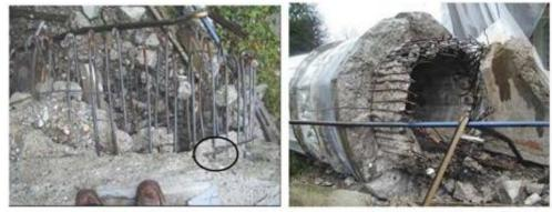
Splicing of Transverse Reinforcement and Hook Ends
