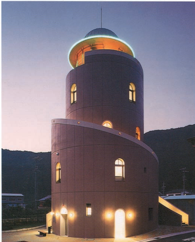
Figure 5-1 Tsunami evacuation structure in Kise, Japan, that includes an archival library on a lower level. A structure such as this can also be used as a community center and may bring in revenue that can be used to repay costs or maintain it.
