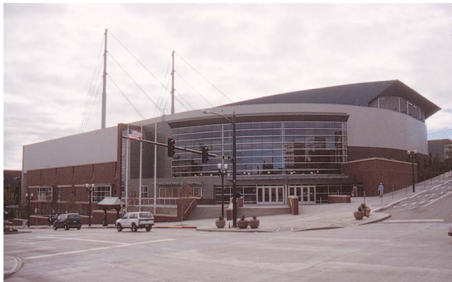
Figure 4-4 Photo of an example sports complex. Facilities of this type, which hold large numbers of people, can serve as a vertical evacuation structure from tsunamis.
