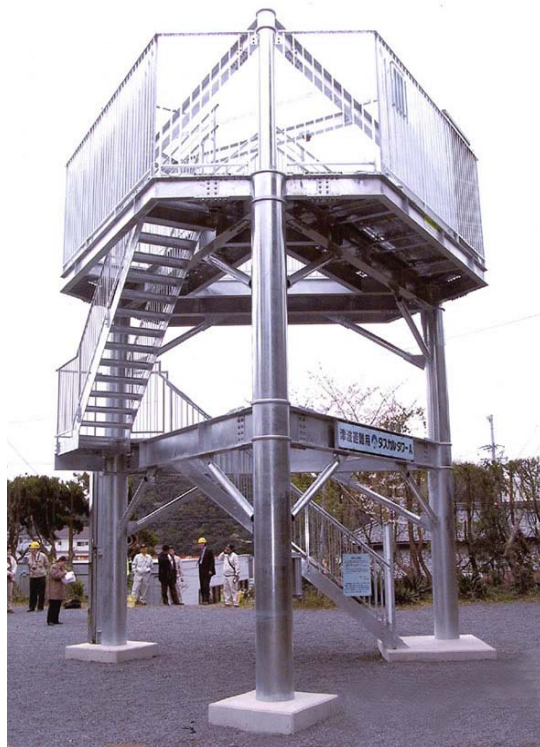
Figure 4-1 Photo of a vertical evacuation structure in Japan that was developed as a simple and economical vertical evacuation option.
