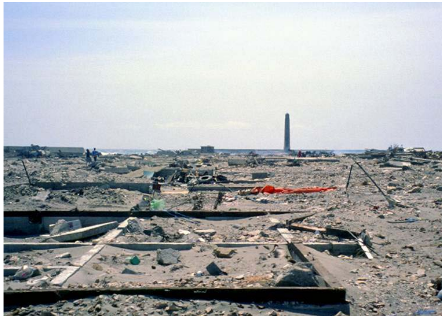
Figure 2-1 Total destruction of a group of wood-frame houses in Aonae Village, Okushiri Island, Japan in the 1993 Okushiri Tsunami.
