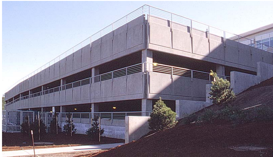
Figure 4-3 A typical parking structure. The design of a parking garage offers some advantages as a vertical evacuation structure.
