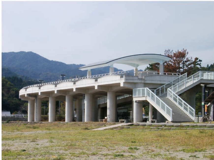
Figure 6-3 Vertical evacuation structure at Shirahama Beach Resort in Japan that is designed as a simple platform to keep people safe during a tsunami.
