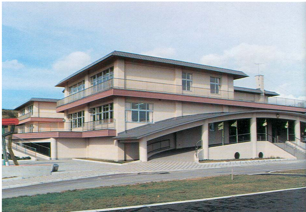
Figure 4-6 School building in Aonae, Japan, in which the upper floors are intended to be used as tsunami refuge space.
