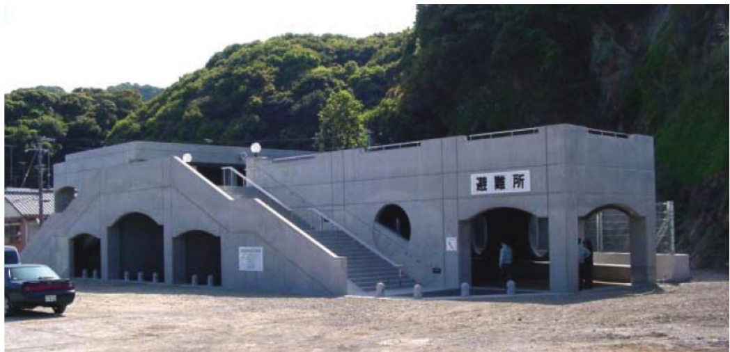
Figure 6-1 A concrete structure in Kaifu, Japan, that is used as a vertical evacuation structure. Structures like this are easy to reach, easy to navigate within, and still provide protection from the destructive forces of tsunamis.
