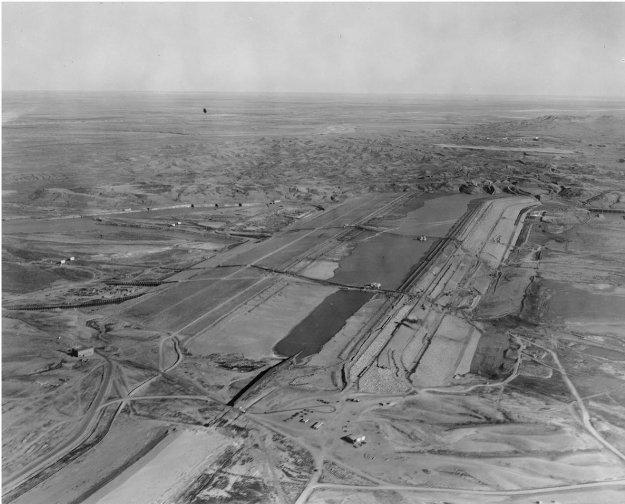
Figure 6. Aerial view of the dam construction in 1937 shortly after completion of the closure section and diversion through the outlet works tunnels.
