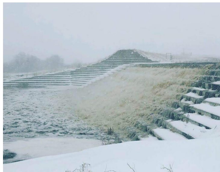
Dam spillway activated during the event
