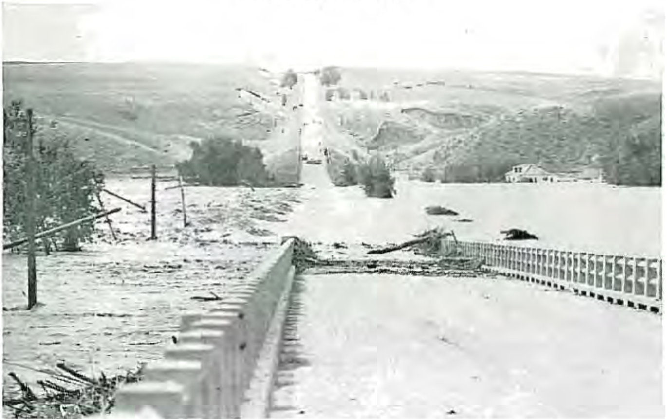
The flood-swollen Marias River at crest early in the week of the flood rose to the level of this Highway 91 bridge south of Shelby in north central Montana, expanded beyond the bridge's end and ran rampant over the earth fill between the bridge end and the highway's incline. Clem Dolven photo.
