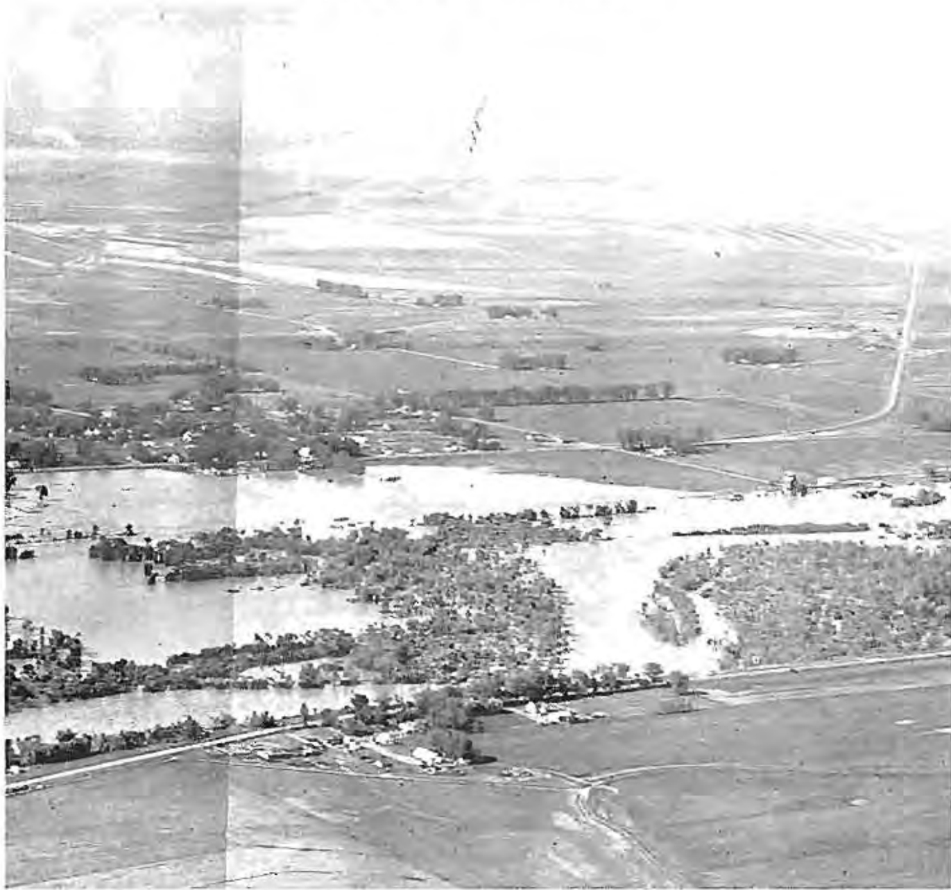
The town of Simms, a small town 30 miles west of Great Falls on the Sun River, was still above water, but the railroad track, center, was flooded and the elevator was surrounded by water. Road to Lincoln and Missoula angles off at right. Air Guard photo.
