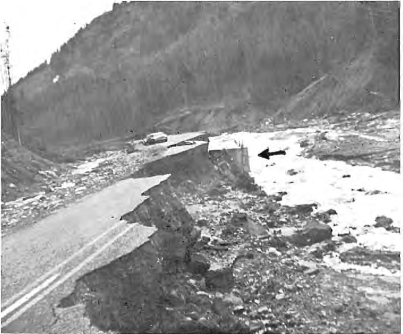
A Helprey truck (arrow), Spokane, became a flood victim when the Middle Fork of the Flathead River washed away Highway 2. Dave Brown, Kalispell, possibly saved the lives of other drivers when he crawled across suspended railroad tracks and reached Summit, where he called for a helicopter. George Goggins photo.
