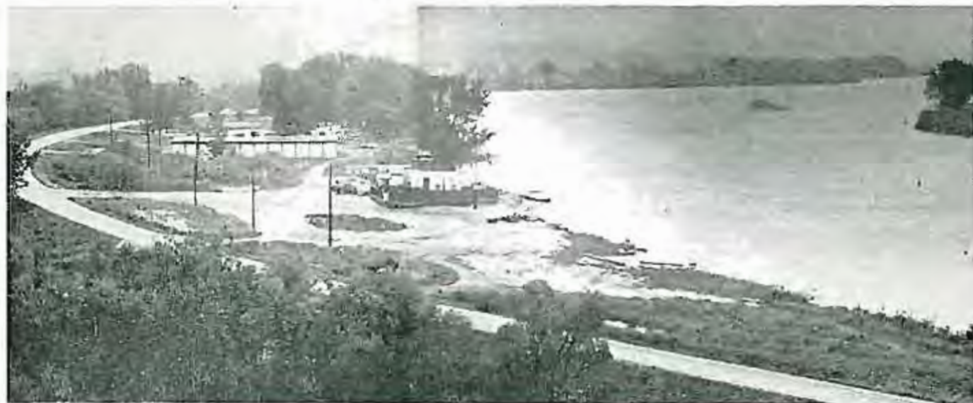
About four miles south of Great Falls, the Missouri River slopped over onto lowlands. Here the water crept up higher later, inundating a number of homes but never covering the highway. Closer to the city, water edged over the highway in several places and seeped into a few more homes and trailer houses. Tribune photo.
