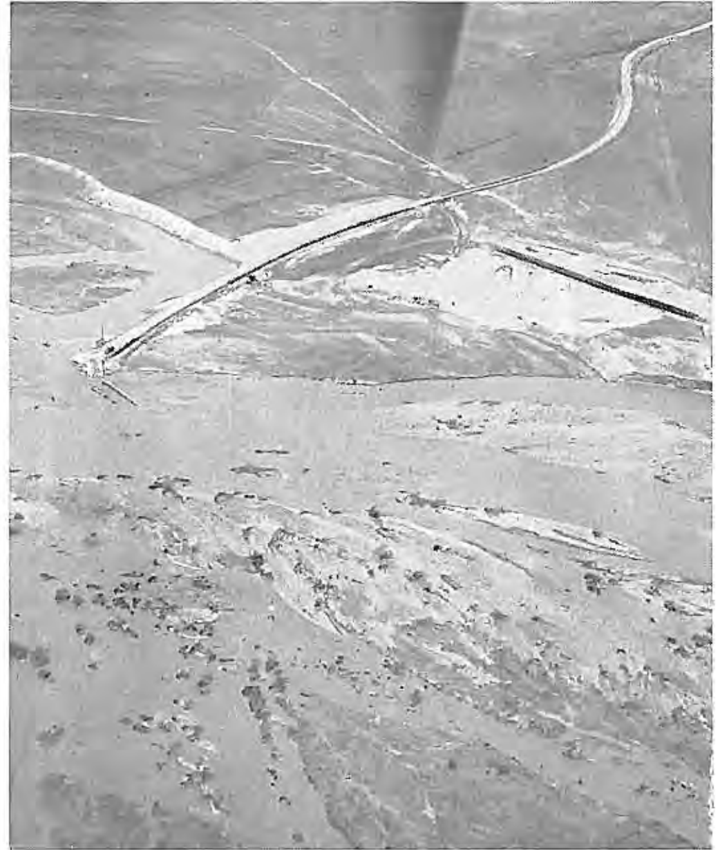
While the river connecting the two St. Mary lakes in Glacier Park stayed in its channel, a small creek near the town of St. Mary ran wild, eroding away a large part of the highway. Tribune photo.
