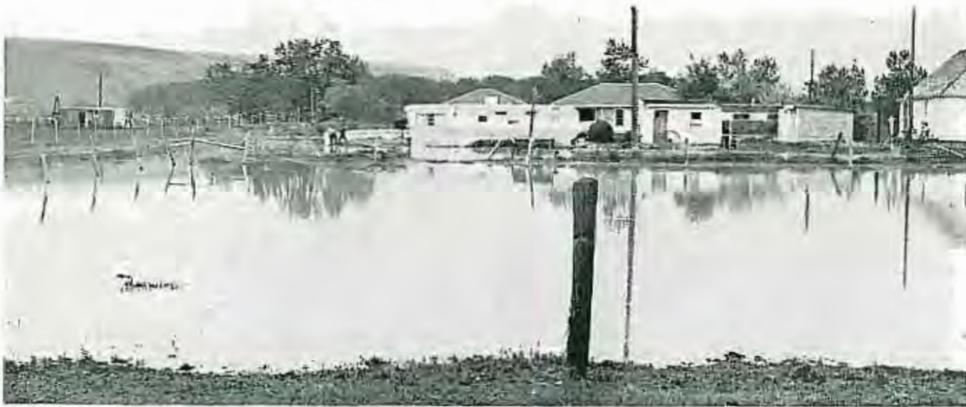
Even before the waters of the Sun River deluged West Great Falls, heavy rains caused the drainage ditch in the foreground to overflow, nearly flooding the house. Tribune photo.
