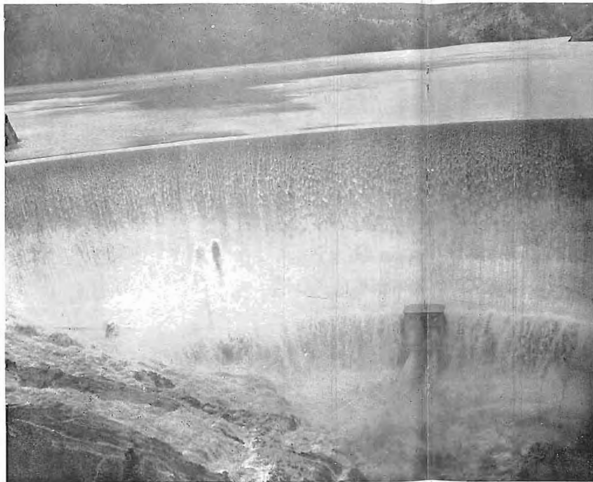
CLOSEUP VIEW OF GIBSON DAM RESERVOIR, OVERFLOW INTO SUN RIVER
