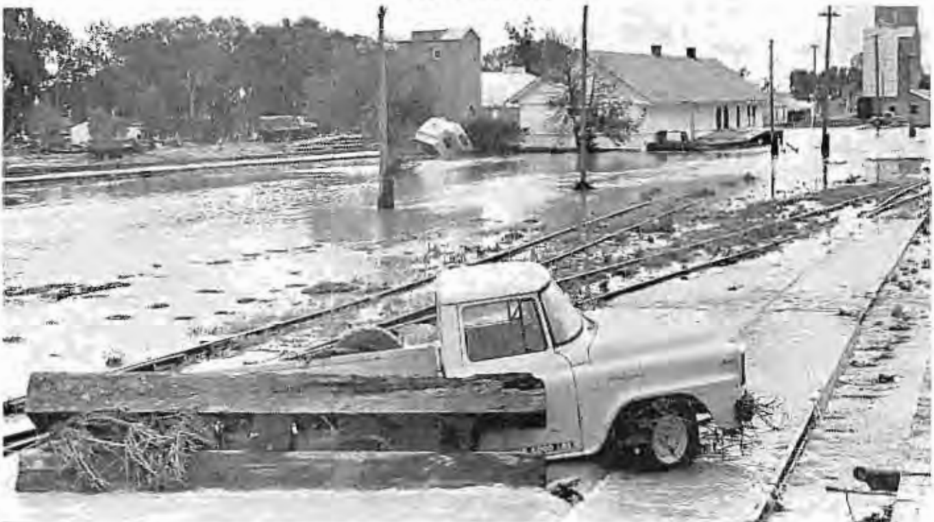
Water rushing through the streets of Choteau wedged this pickup truck against the railroad tracks in the downtown section. This area was in the hardest hit part of town. AP Photofax.
