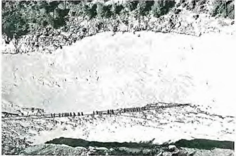
The flooded, silt-laden Middle Fork of the Flathead River destroyed this stretch of Great Northern Railway track between West Glacier and Essex. Guest photo.
