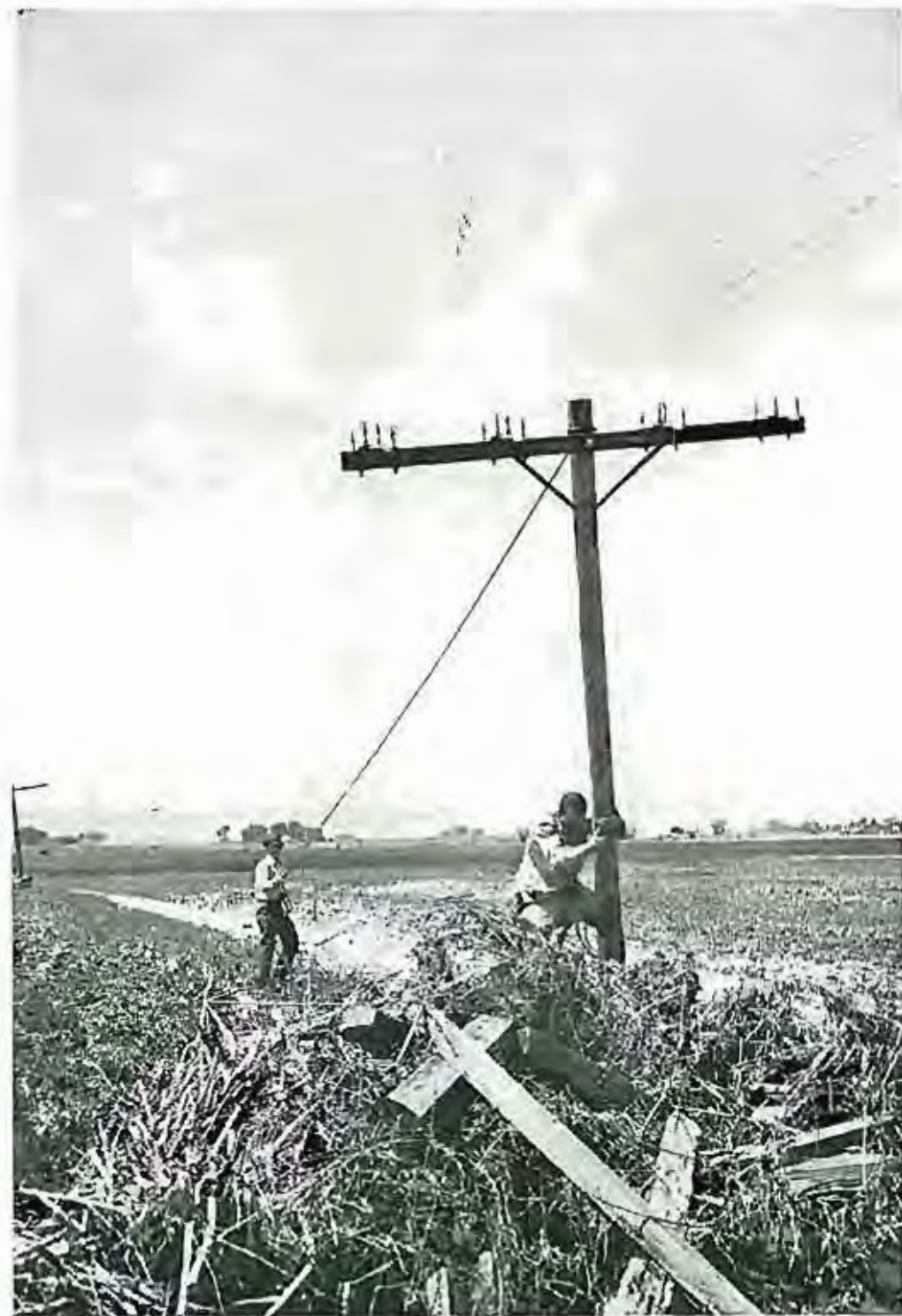
Telephone crews near Sun River work to restore service after the flood in a battle with debris and broken poles. Mountain States Telephone photo.
