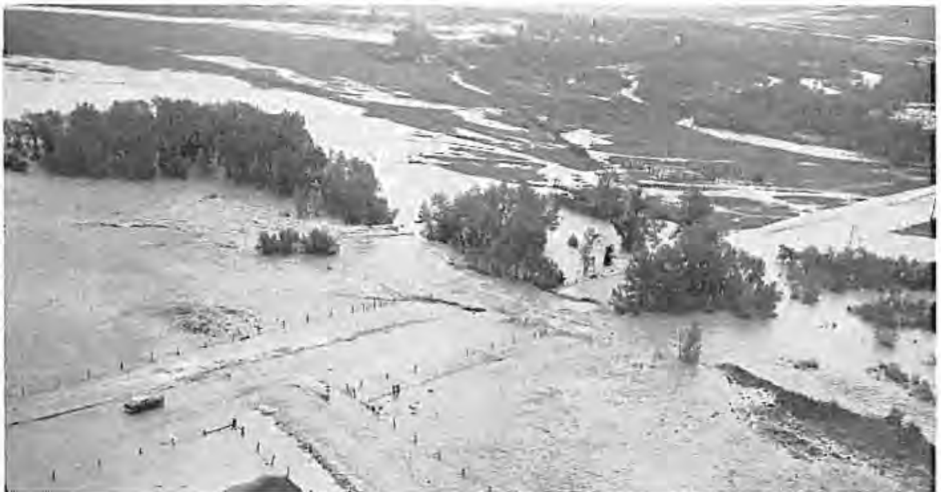
Swollen torrents in the Dupuyer area in Pondera County knifed through this stretch of road and stranded a motorist whose car is at left. DeMier photo.
