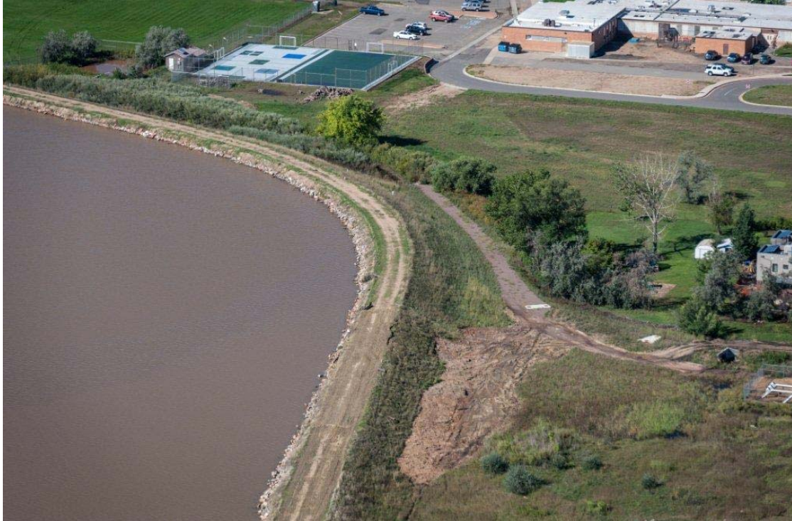
Figure 8 - Aerial photo of the Baseline Northwest dam with temporary stabilization measure in place and a declining reservoir level.
