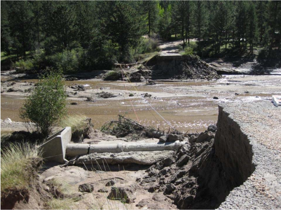
Figure 6 - Photo of the Rainbow Lake dam breach taken on September 25, after 12 days of continuous high flows.
