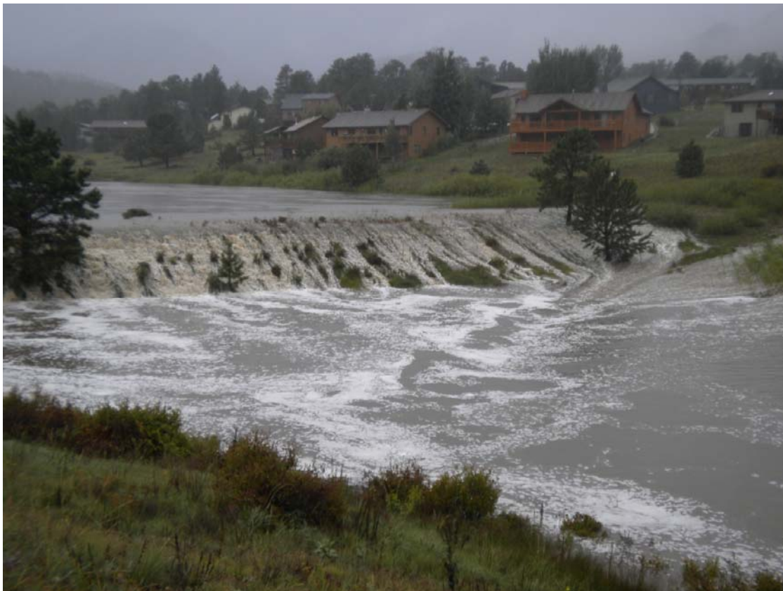
Figure 9 - Photo of Carriage Hills No. 1(upper dam) overtopping taken on Thursday September 12, 2013 by an Estes Park resident.
