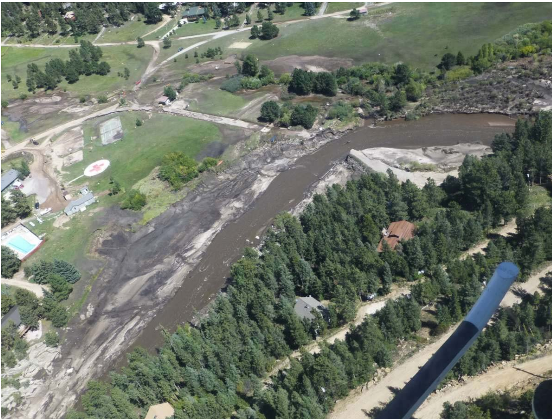
Figure 5 - Photo of main access to Big Elk Meadows subdivision over the Mirror Lake dam, taken from the air on September 17..
