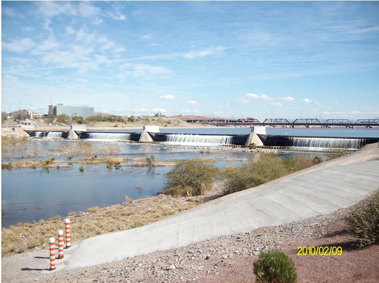
**Figure 1.** Tempe Town Lake Dam with four (4), 16-foot high, 200-foot long rubber bladders forming a lake within the Salt River banks in Arizona prior to failure
