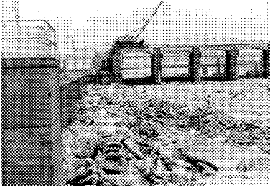
Figure 7. Accumulation of broken ice upstream of Lock and Dam 26, 11 February 1966, Alton, Illinois.
