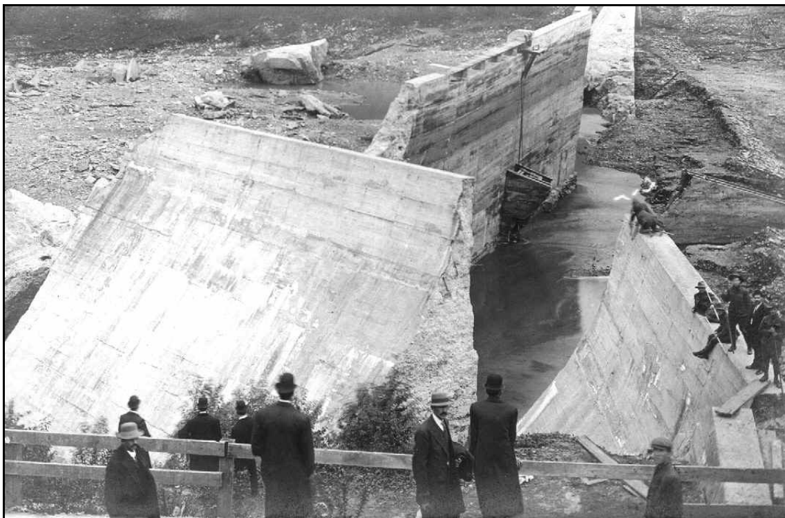
Figure 5. Catastrophic Collapse, September 30, 1911 (Source: Potter County Historical Society).
