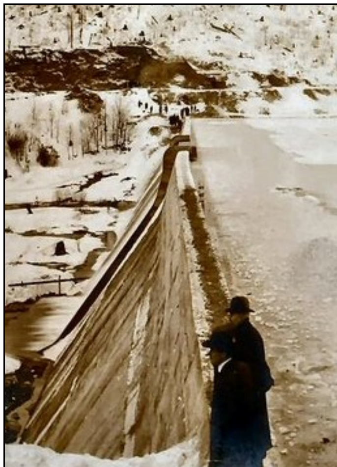
Figure 3. Partial Sliding Failure, January 23, 1910 (Source: Potter County Historical Society).
