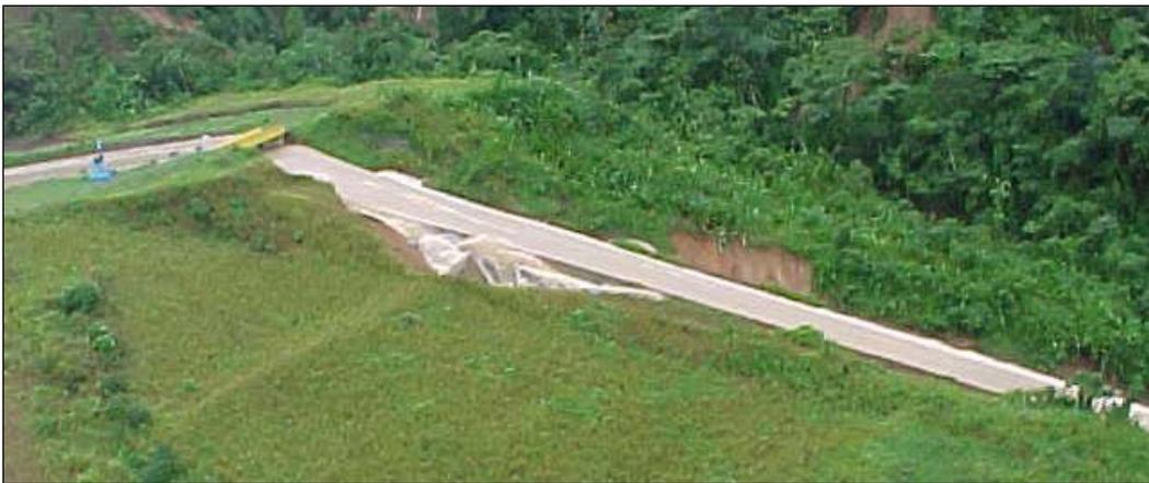
Figure F-2-9.—Overtopping along entire length of chute.
