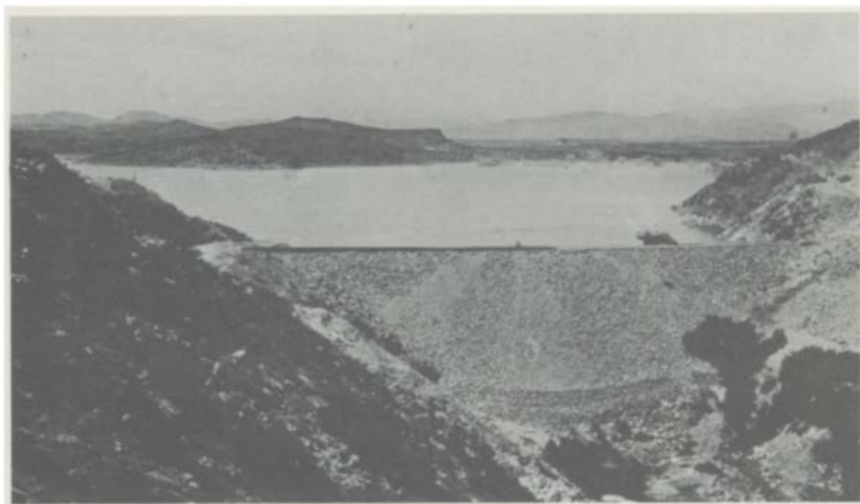
Figure 2. Photo of Walnut Creek Dam and Reservoir (Dill (1987), The Walnut Grove Dam Disaster of 1890, The Journal of Arizona History ).
