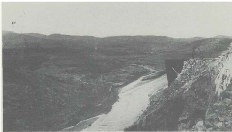
Figure 3. Photo of remnant of Walnut Creek Dam after failure (Dill (1987), The Walnut Grove Dam Disaster of 1890, The Journal of Arizona History).
