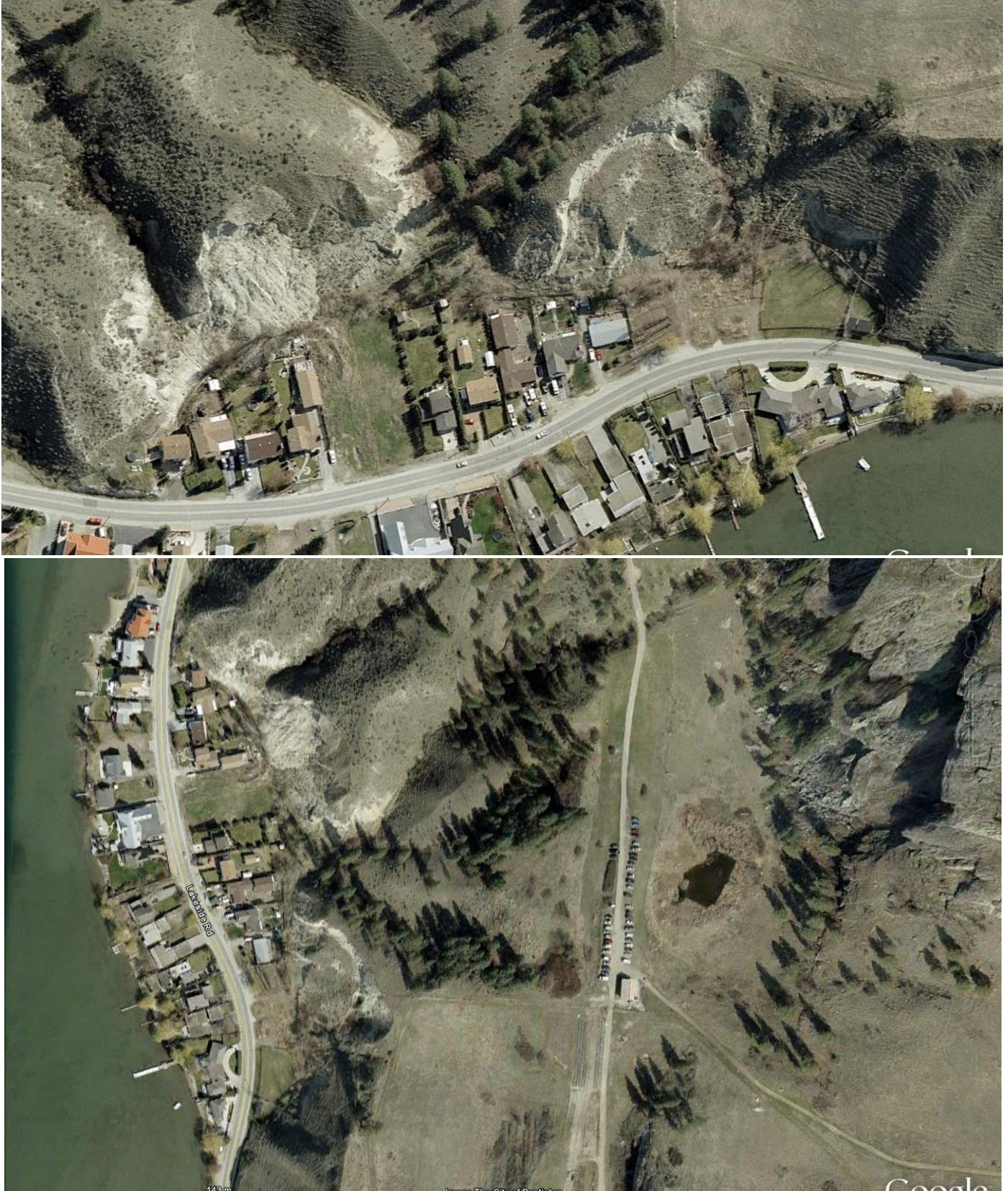
Figure 18. Aerial views of Lakeside Road landslides.
