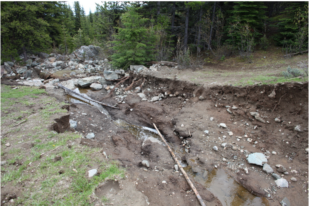
Figure 27. Downstream face of dam breach.
