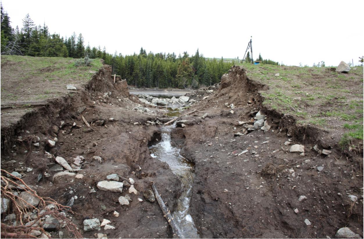
Figure 26. Testalinden lake dam breach.
