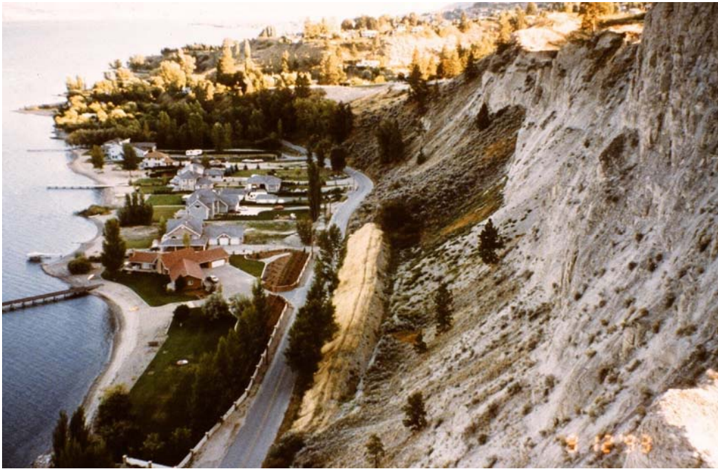
Figure 10. Schuster slide area showing toe berm built after the landslide (N. Skermer).
