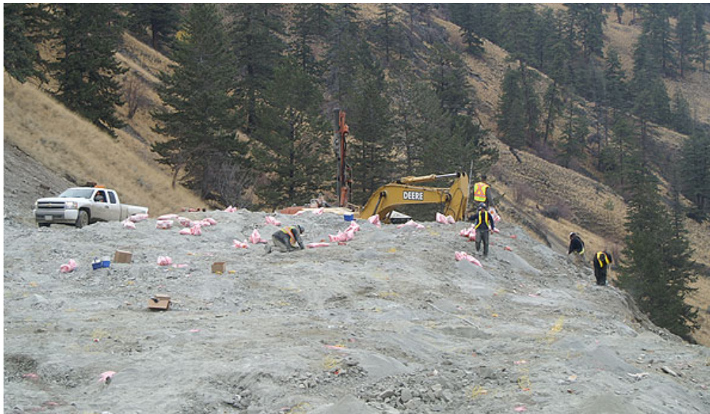
Figure 7. Preparation for removing 17,700 m 3 of rock (Arthon Construction, Oct. 2008).
