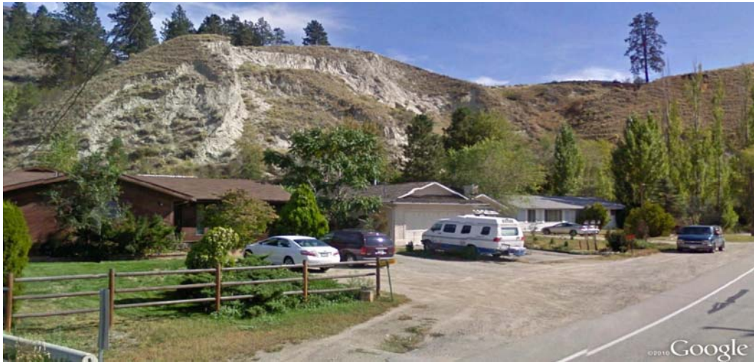
Figure 19. Google Streetview images of Lakeside Road landslides.
