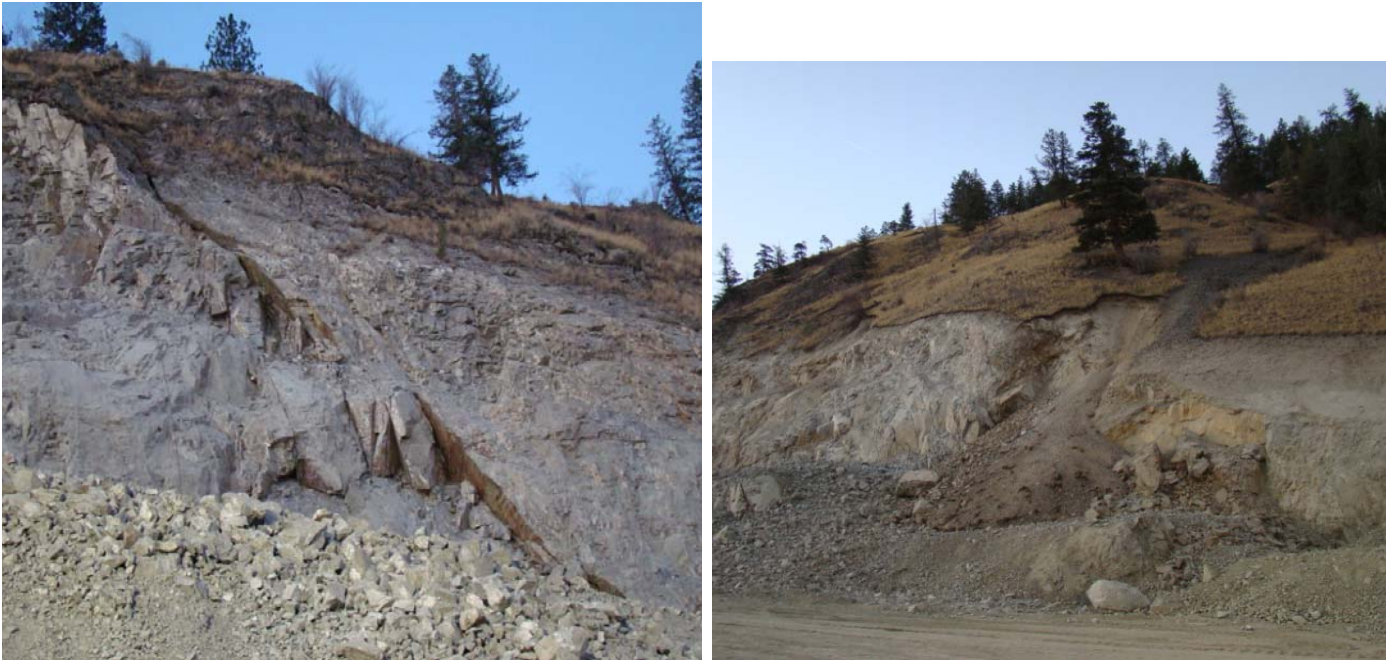
Figure 4. Slope movement along slip surface (day-lighted portion - left, buried under colluvium - right).
