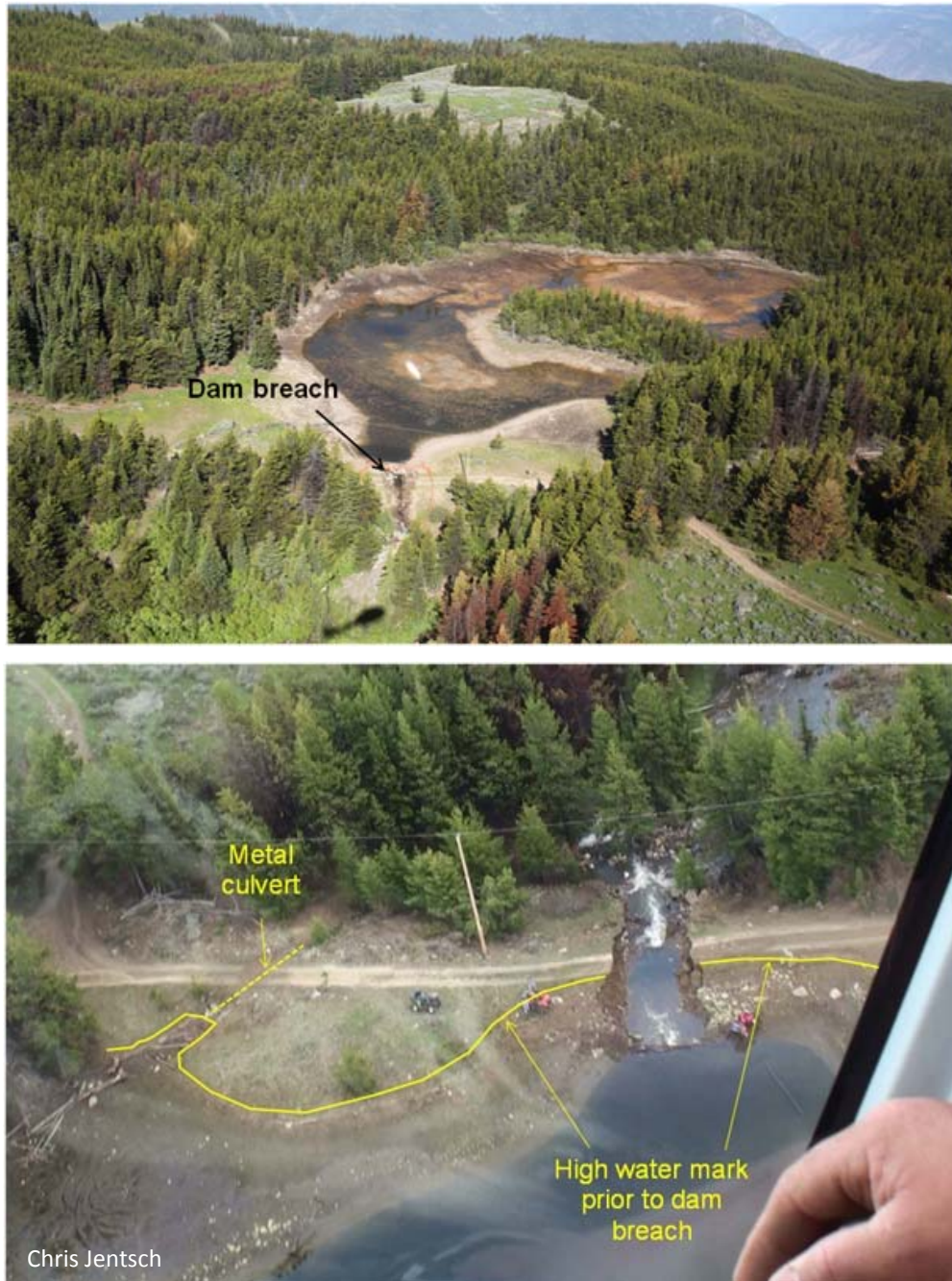
Figure 25. Testalinden lake dam breach.
