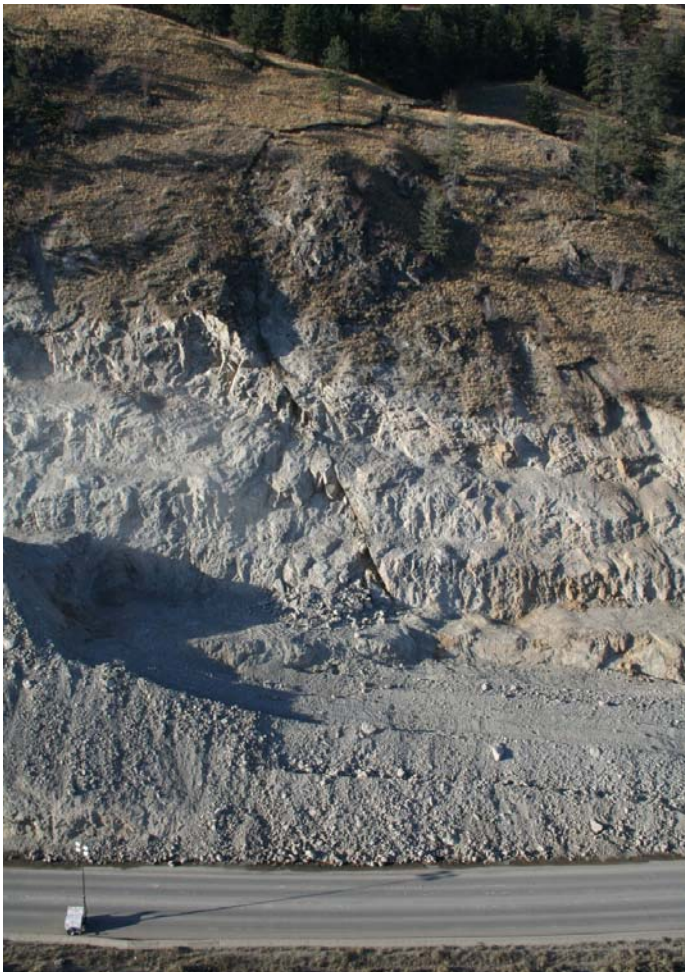
Figure 3. Tensile fracture and slip surface (Arthon Construction, Oct. 2008).
