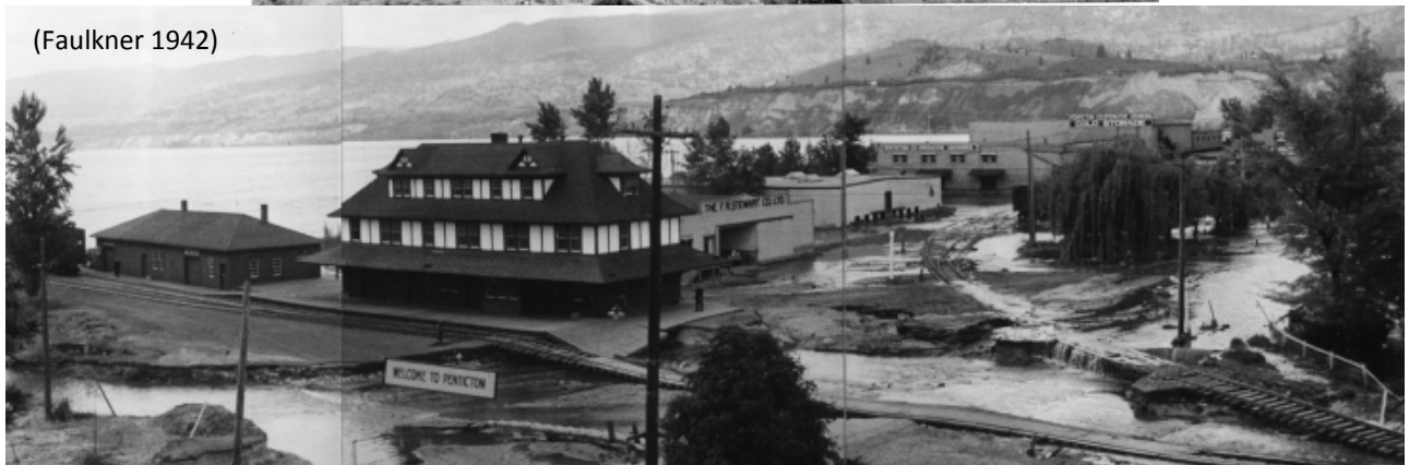
Figure 21. Dam failure at wooden spillway in 1942 and flood in Penticton.
