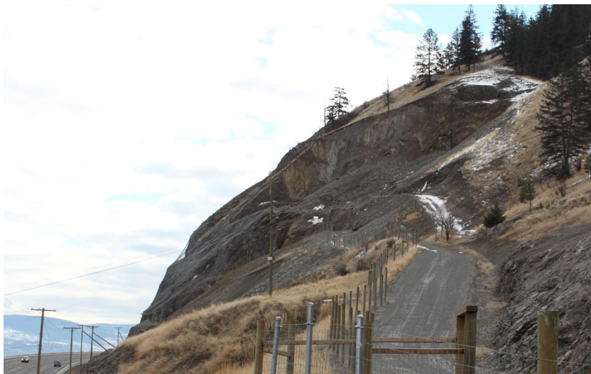
Figure 8. Completed construction with upper part of slope above the slip surface removed.
