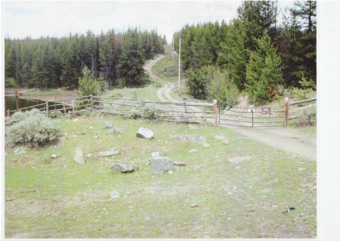
Testalinden Lake and Dam, June 2009
