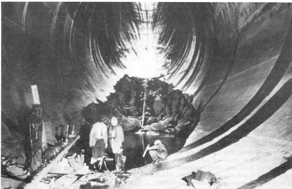
FIGURE 7-7.—Hoover Dam, Arizona tunnel spillway — major damage (1942).
