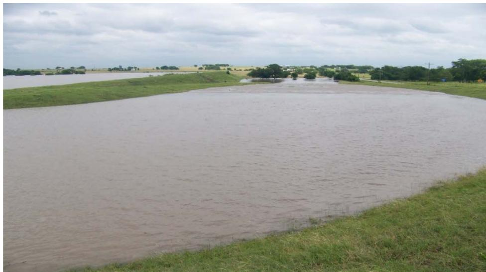
Figure 6: Auxiliary spillway functioning as designed
