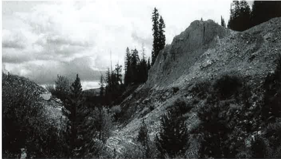
Figure 5: Remnants of Dam in 2002 Looking Upstream Note: Left Abutment Spillway Channel at Top Right in Photo
