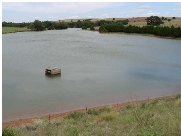
Existing principal spillway inlet on Sugar Creek Watershed Dam No. L-43.
