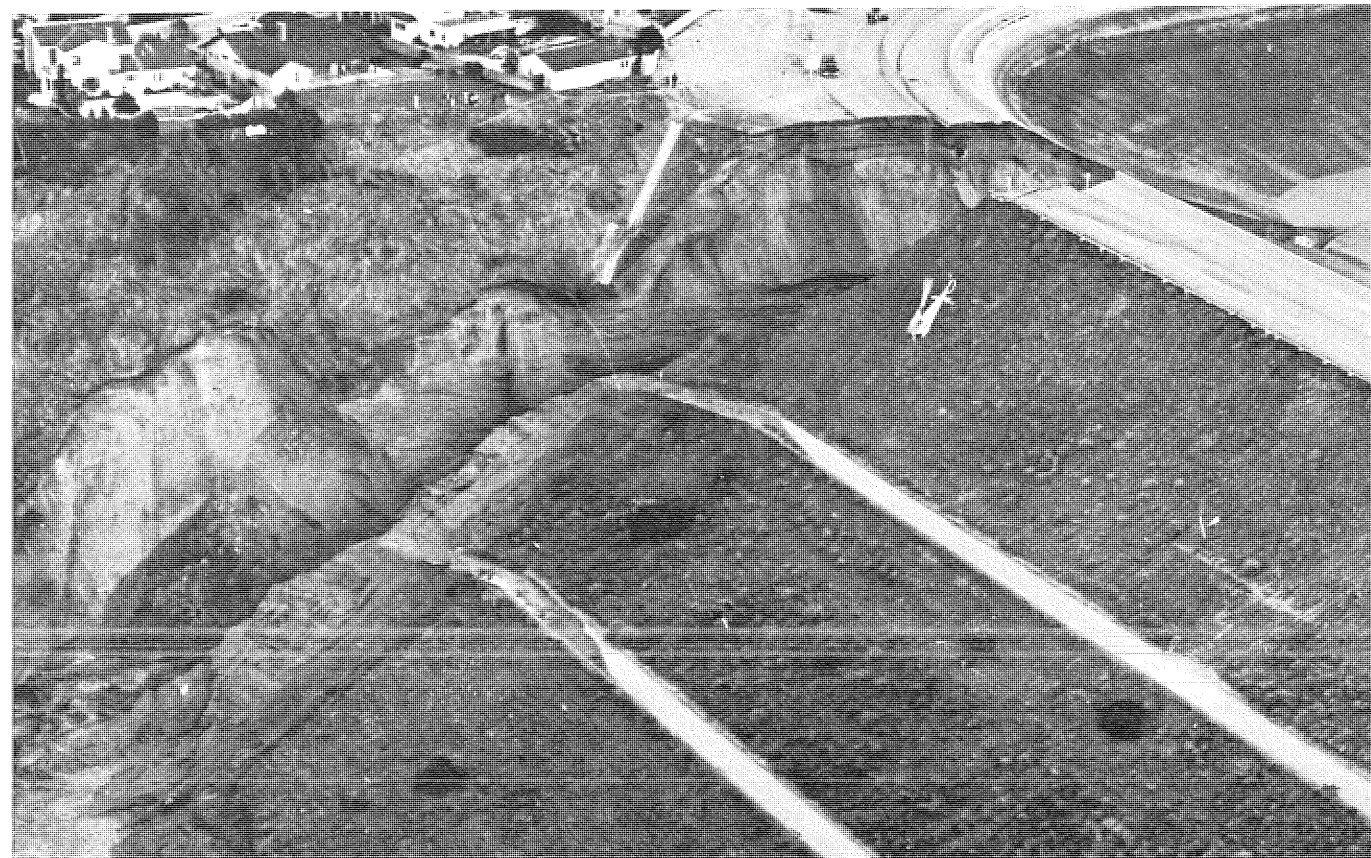
PHOTO 16. Breach with failure complete and reservoir almost empty.
