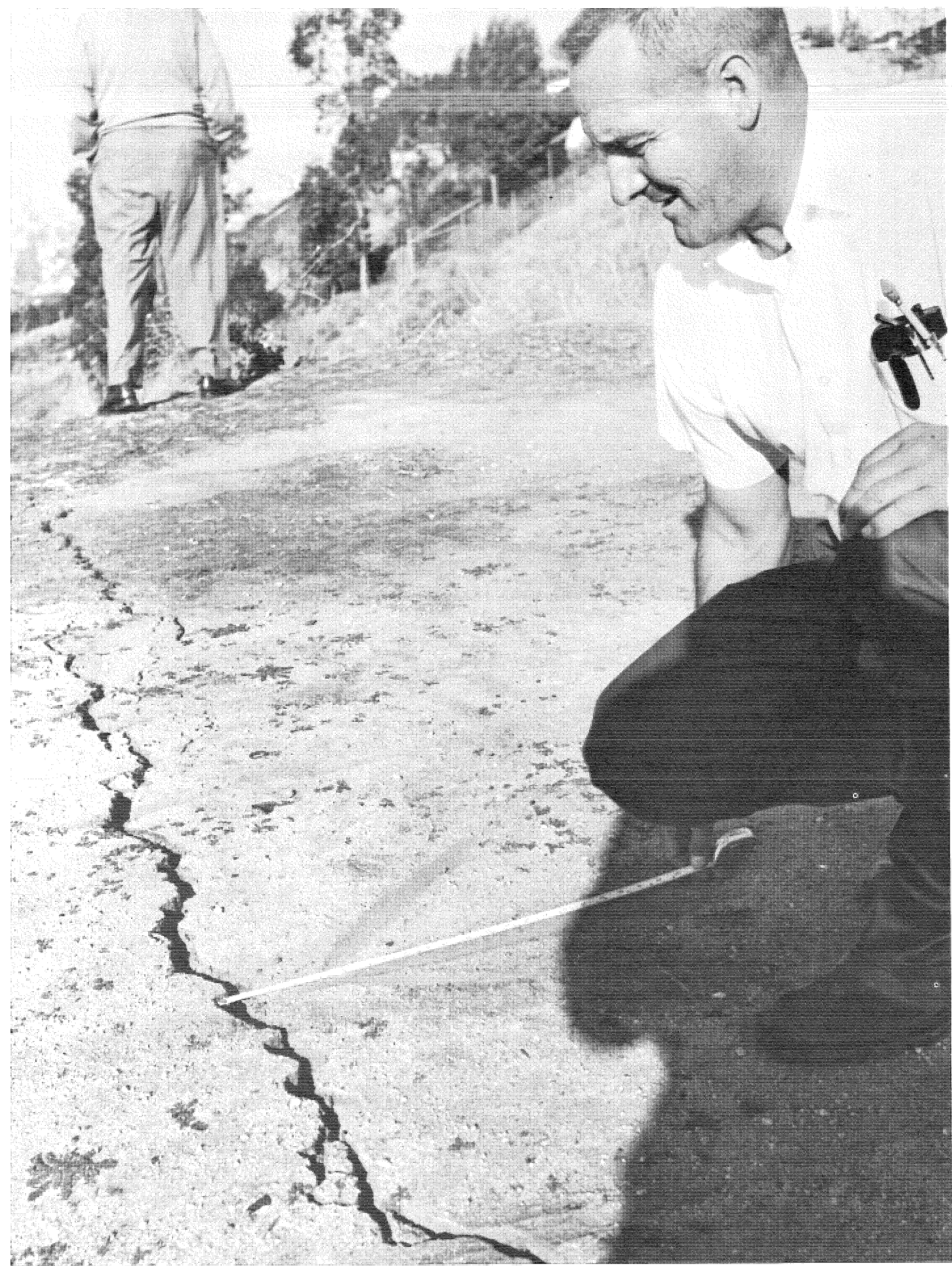
PHOTO 13. Crack at crest of main dam near east abutment.
