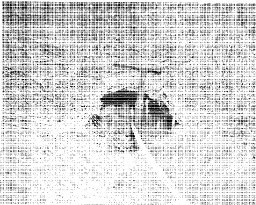
PHOTO 54. Earthcrack 2 near northwest corner of Stocker Street and La Brea Avenue, showing pothole which is typical of this type of earthcrack.
