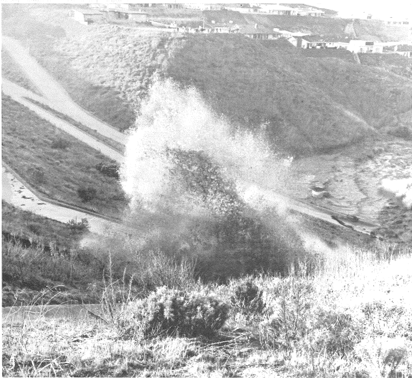
PHOTO 4. Flow through breach during final stage of failure, at about 4:00 p.m. Spray caused by material falling into flow.
