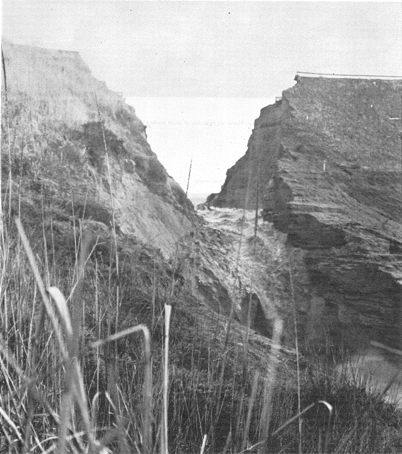
PHOTO 14. Discharge following dam crest collapse, at approximately 3:40 p.m.
