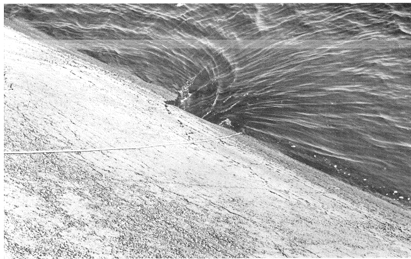
PHOTO 5. Discovery of hole on face of main dam at approximately 2:20 p m.
