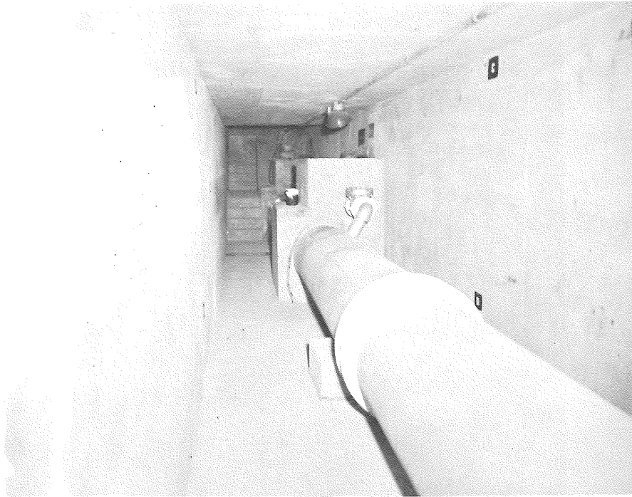
PHOTO 47. Drainage inspection chamber, January 10, 1952, showing 24-inch blowoff pipe in foreground and weir box for southeast toe, northeast toe, and fault drains in rear. Labels C and D on south wall locate crack at Station 0+70.3.
