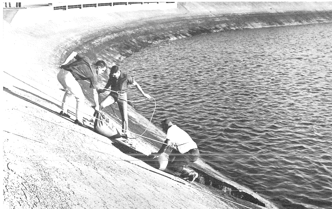
PHOTO 6. Attempt at sandbagging hole in main dam, at about 2:50 p.m.
