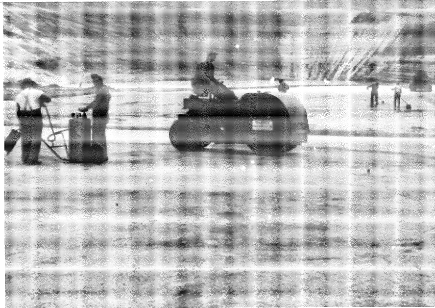
PHOTO 33. Rolling loose pea gravel into asphaltic membrane.
