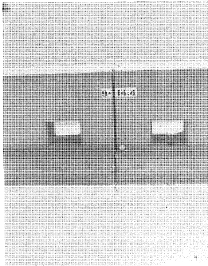
PHOTO 52. Opening in north parapet wall at Station 9+14.4, May 16, 1955.
