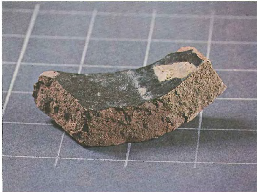
PHOTO 87 Another view of broken clay tile pipe taken from Excavation No. 8.
