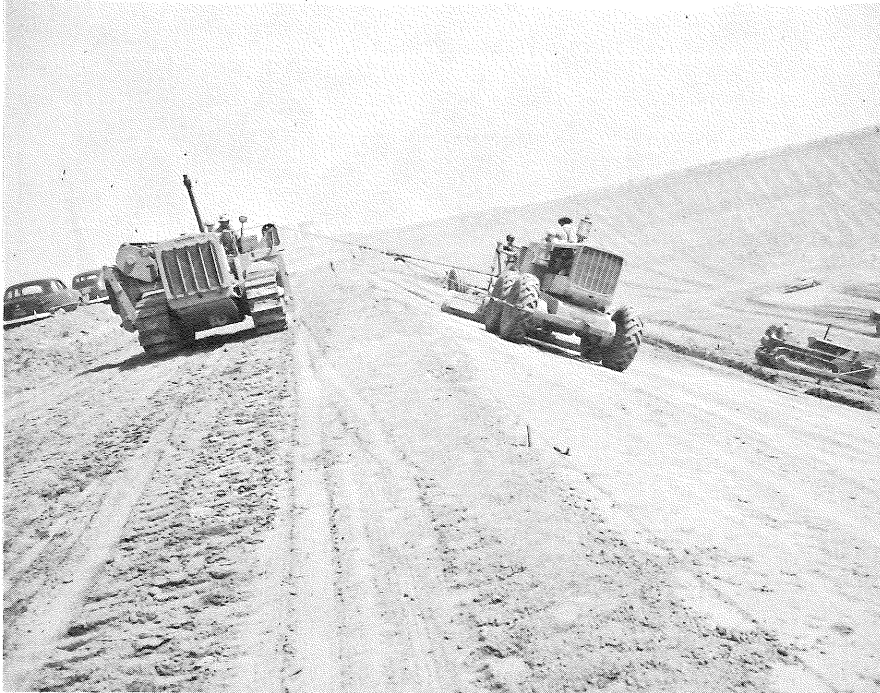
PHOTO 30. Winch tractor and motor grader trimming inside slope.
