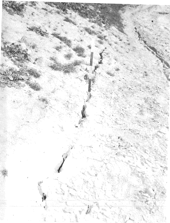
PHOTO 58. Earthcrack 10. Looking north at open eroded crack in south bank of Cloverdale Avenue.
