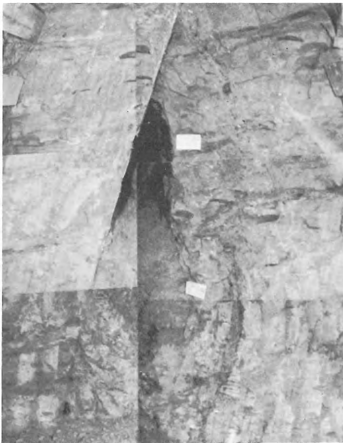
PHOTO 89. Mosaic showing cavity along Fault I at Station 0+62 in Excavation No. 9. Cavity extends beyond face to distance of 4.5 feet.
