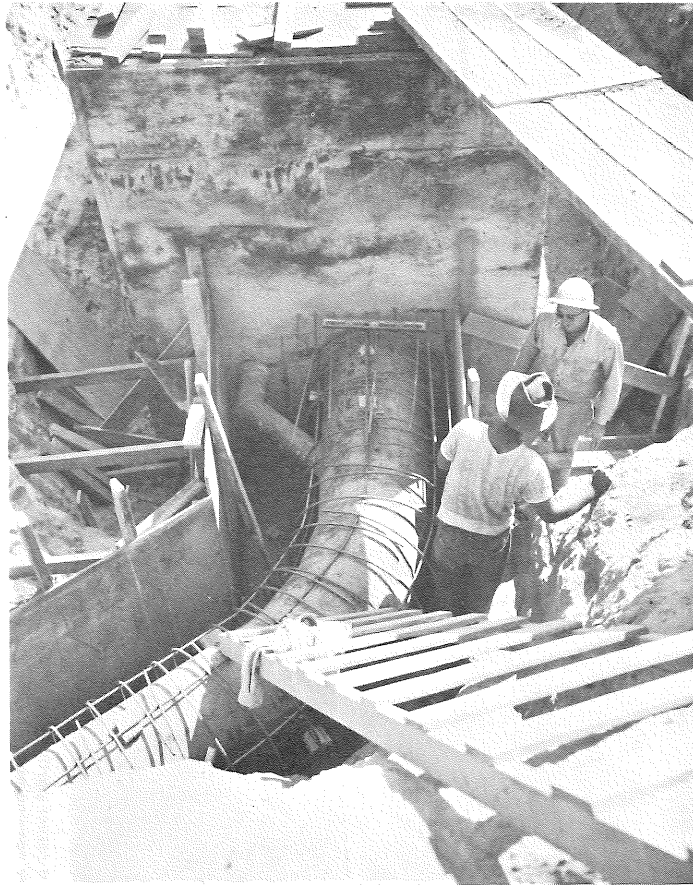
PHOTO 44. Junction of 24-inch blowoff and inspection chamber.
