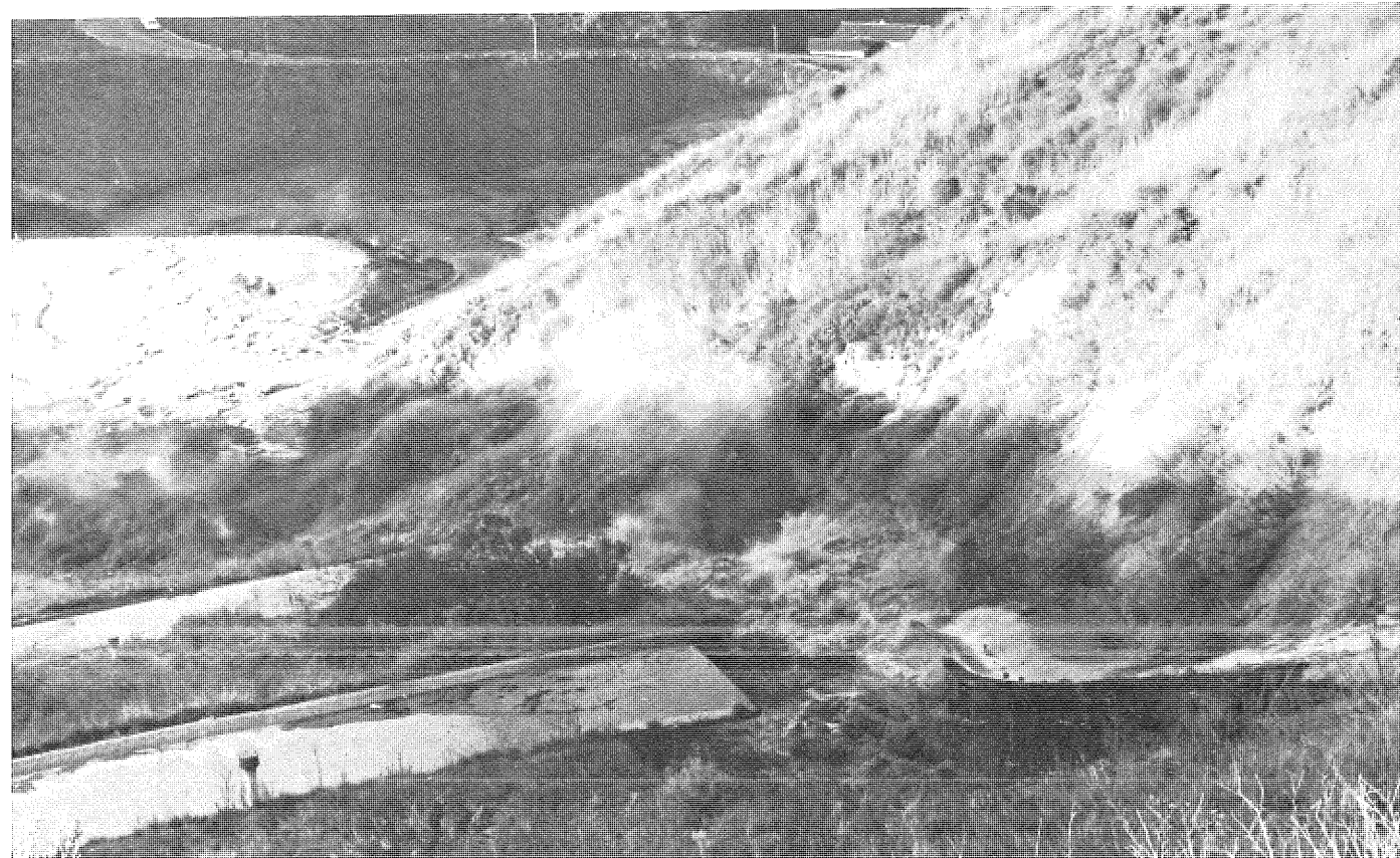
PHOTO 3. Accelerating discharge at about 3:30 p.m. Observe ponding at street embankment.
