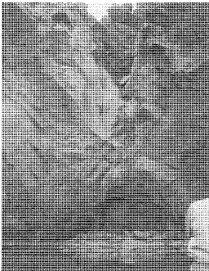
PHOTO 69. Looking upstream at faulted Pico formation in lower end of breach, December 16, 1963.
