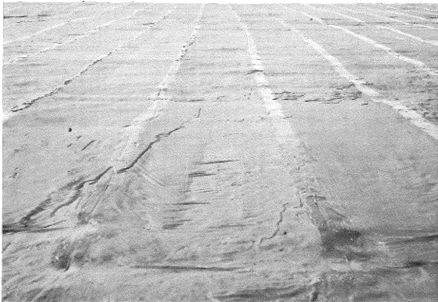
PHOTO 31. Fabric-reinforced asphaltic membrane on west slope.
