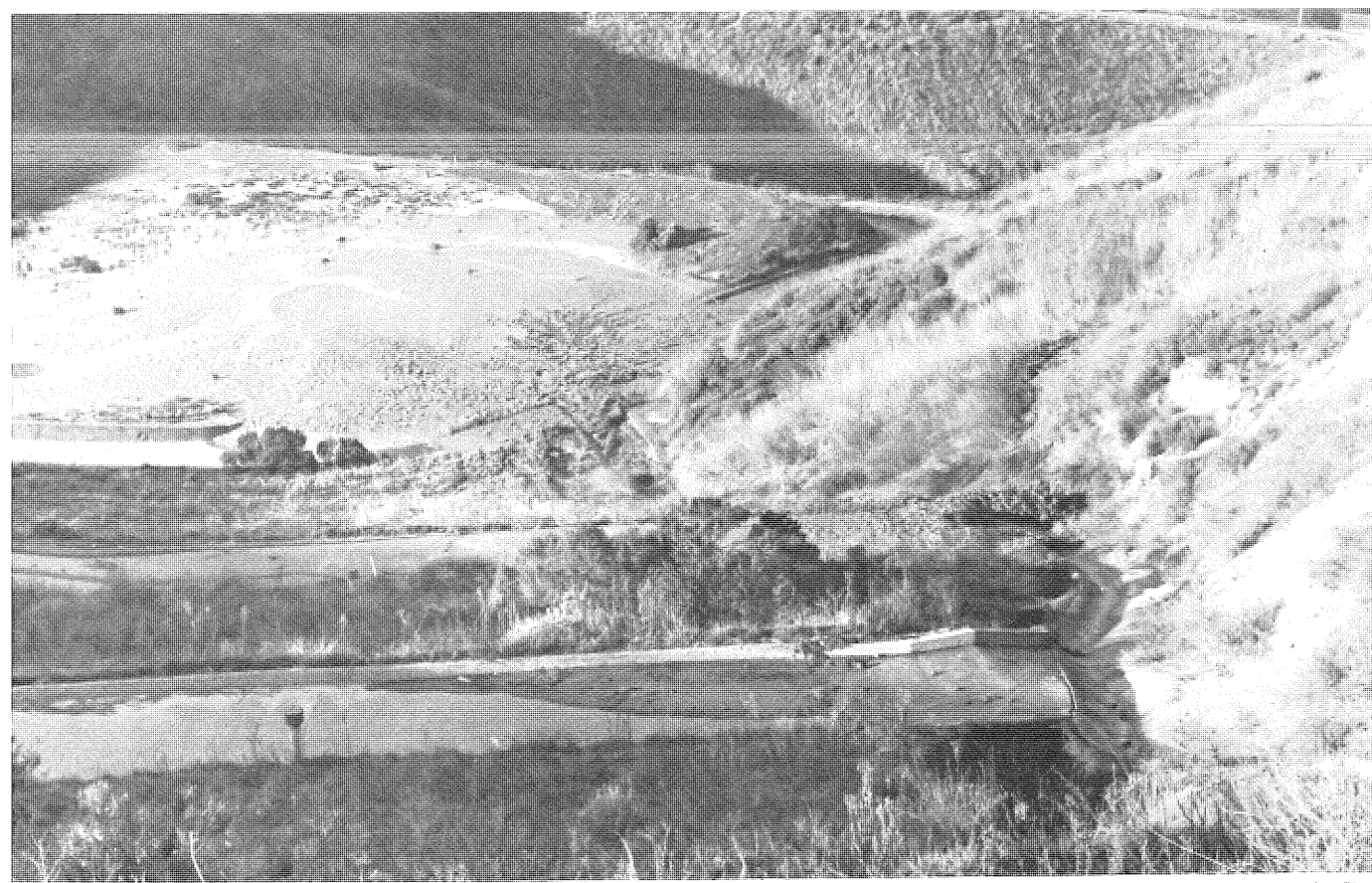
PHOTO 2. Flow spreading on Elevation 340 berm. Estimated time 2:30 p.m. Note submergence of catch basin and cavities developing at gutter.
