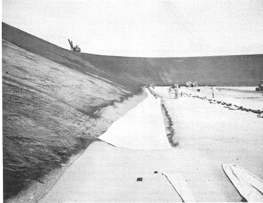
PHOTO 32. West toe drain ditch after placing fabric reinforcing.
