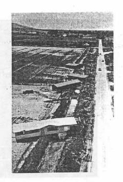
REXBURG, IDAHO—HOUSES MOVED FROM THEIR FOUNDATIONS AS A RESULT OF THE TETON DAM FAILURE
