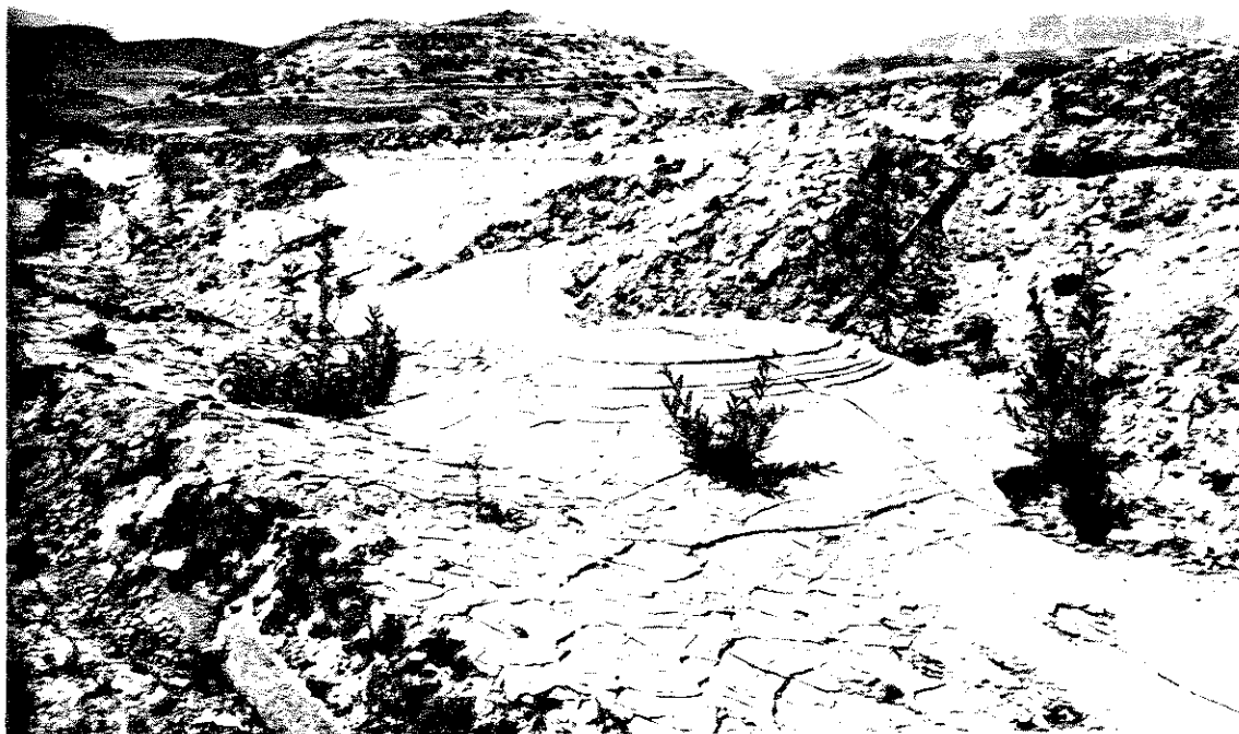
FIG. III-23 SAND BOILS IN THE DEPRESSION SCARPS NEAR THE TOE OF THE SLIDE DEBRIS, LOWER SAN FERNANDO DAM.
