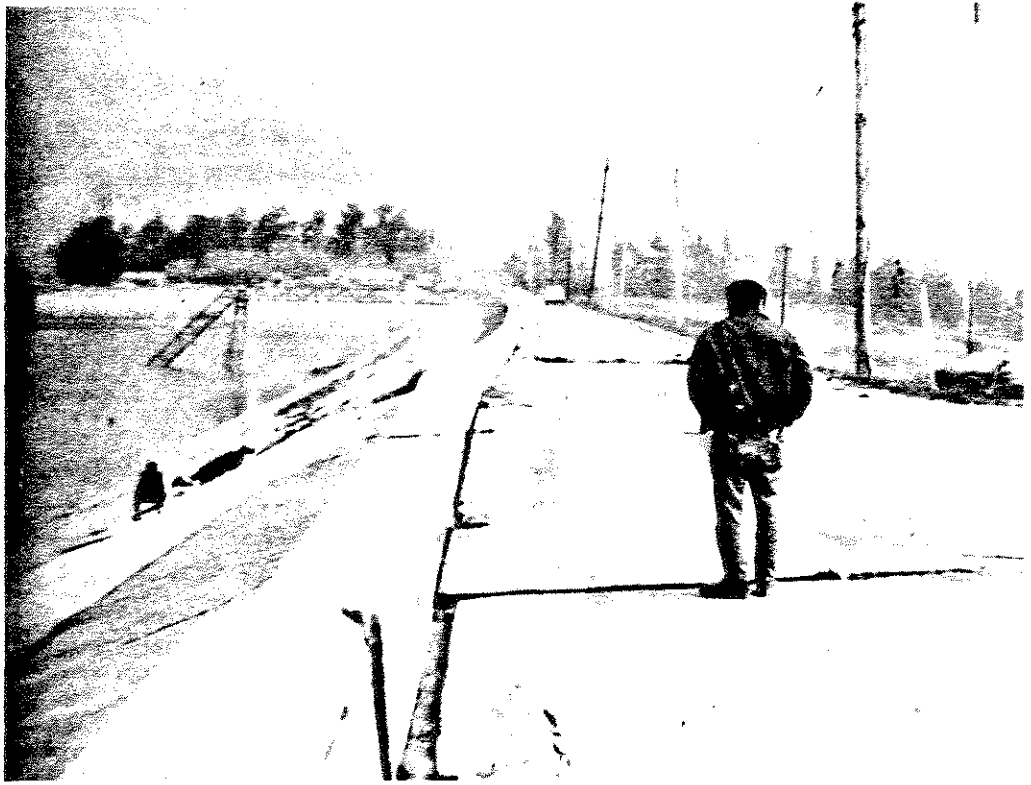
FIG. III-6 DEFORMATION OF PARAPET WALL RESULTING FROM DOWNSTREAM MOVEMENT OF EMBANKMENT
