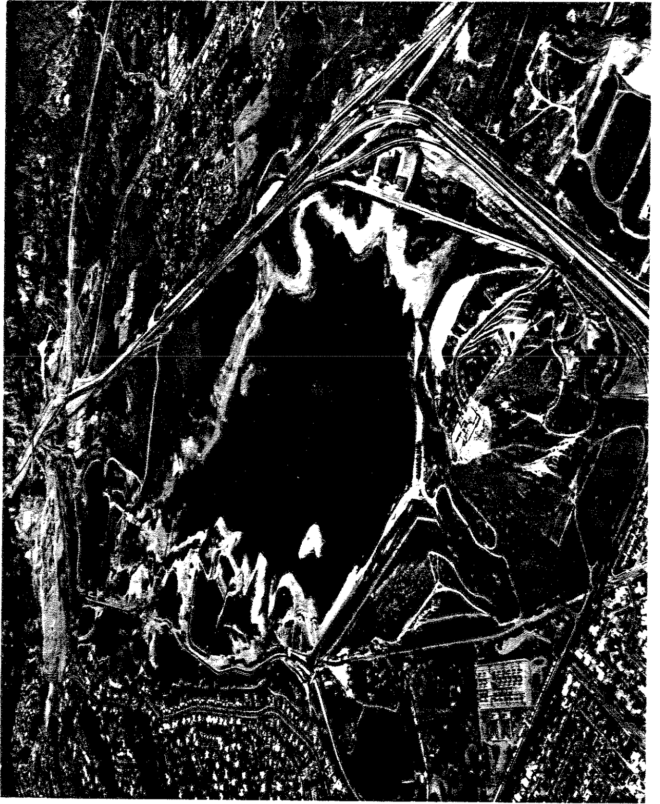
FIG. 1-1 AERIAL VIEW OF VAN NORMAN LAKE COMPLEX TAKEN AFTER EARTHQUAKE. (Photograph by Department of Water Resources)
