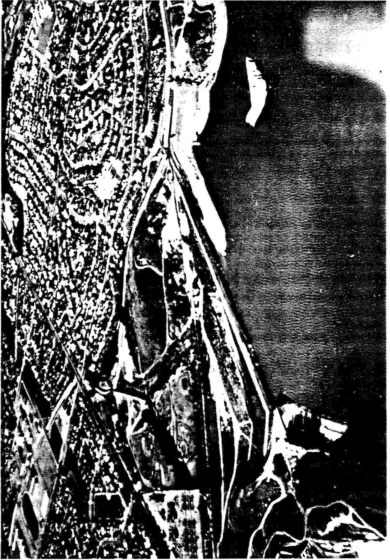
FIG. III-12 AERIAL VIEW OF LOWER SAN FERNANDO DAM SOON AFTER EARTHQUAKE
