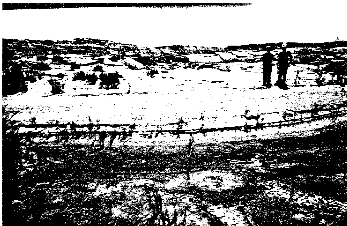
FIG. III-24 TOE OF THE SLIDE DEBRIS, LOWER SAN FERNANDO DAM.
