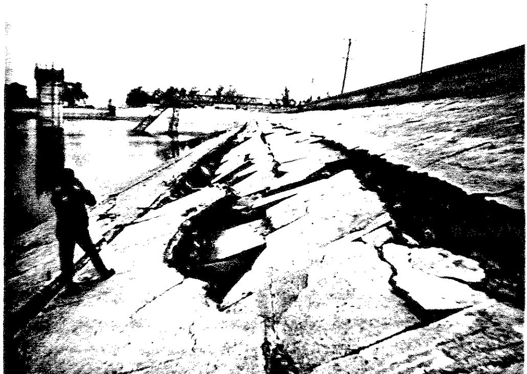
FIG. III-7 SLIDE SCARPS ON UPSTREAM FACE OF EMBANKMENT
