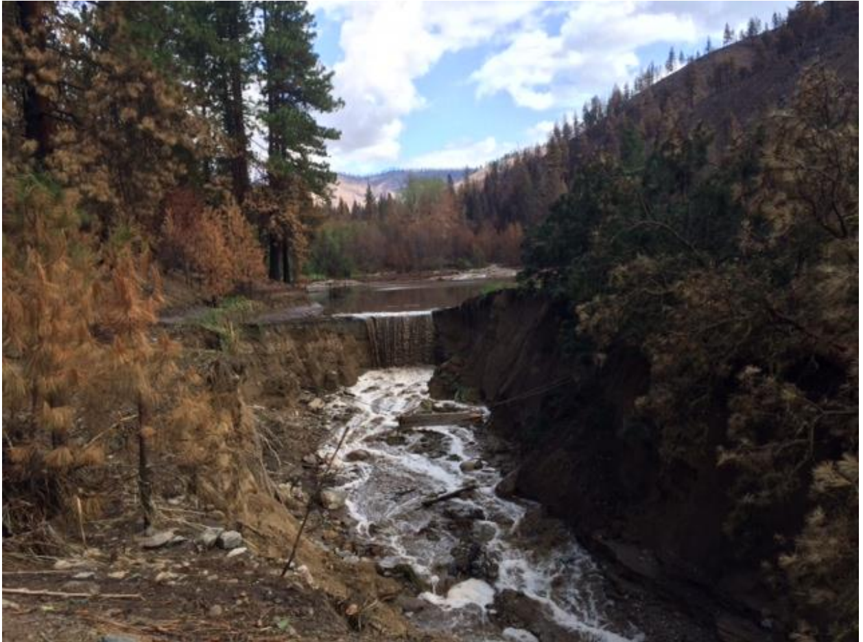
5. Hawkins Dam (Wenner Lake No.5) spillway, mid-day on August 22 nd .
