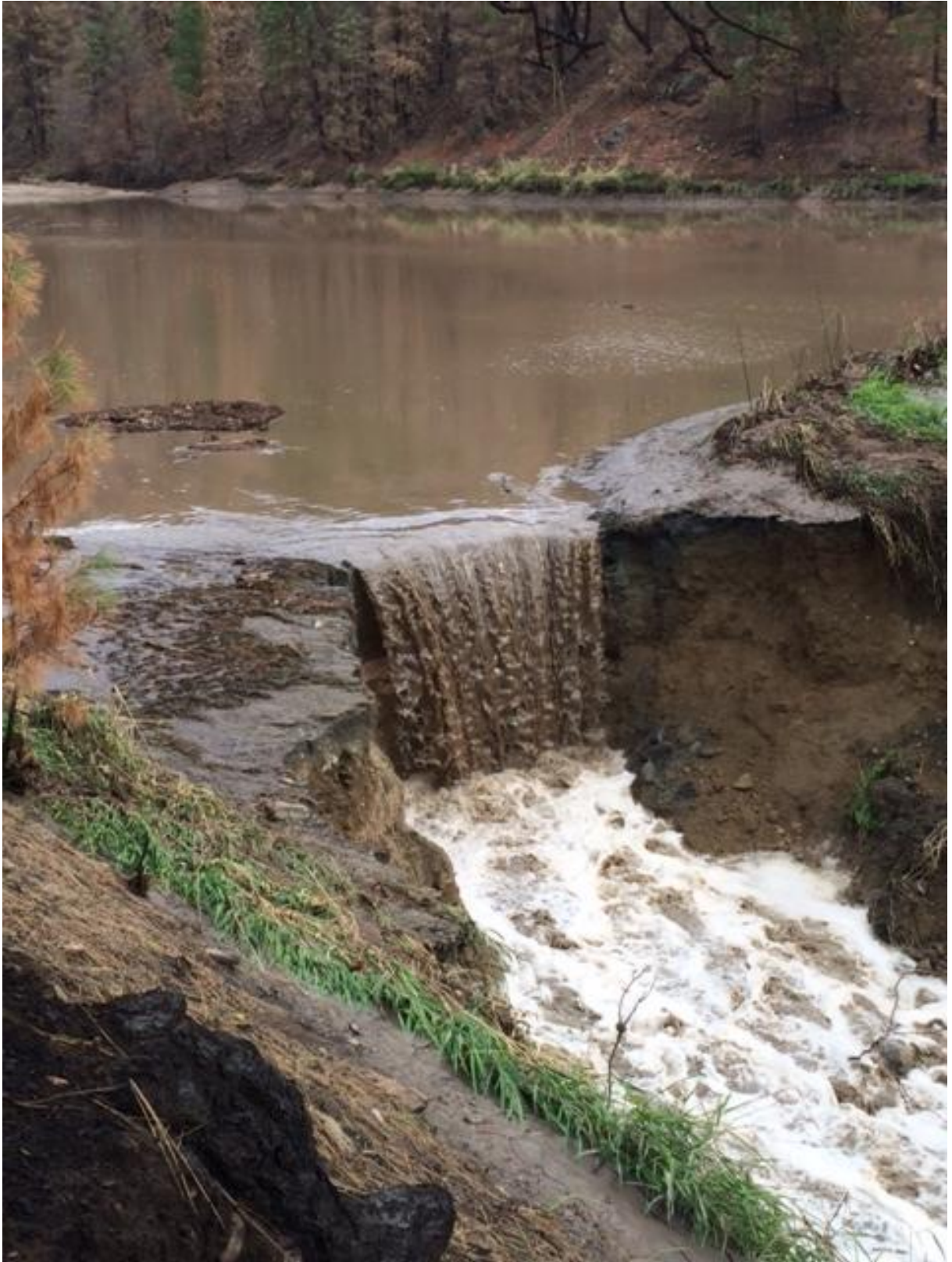
6. Hawkins Dam (Wenner Lake No.5) spillway, mid-day on August 22 nd .
