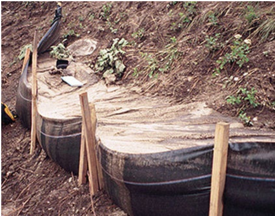
Figure B-6 Fully loaded silt fence placed after the 2000 Bitterroot Valley complex wildfire
