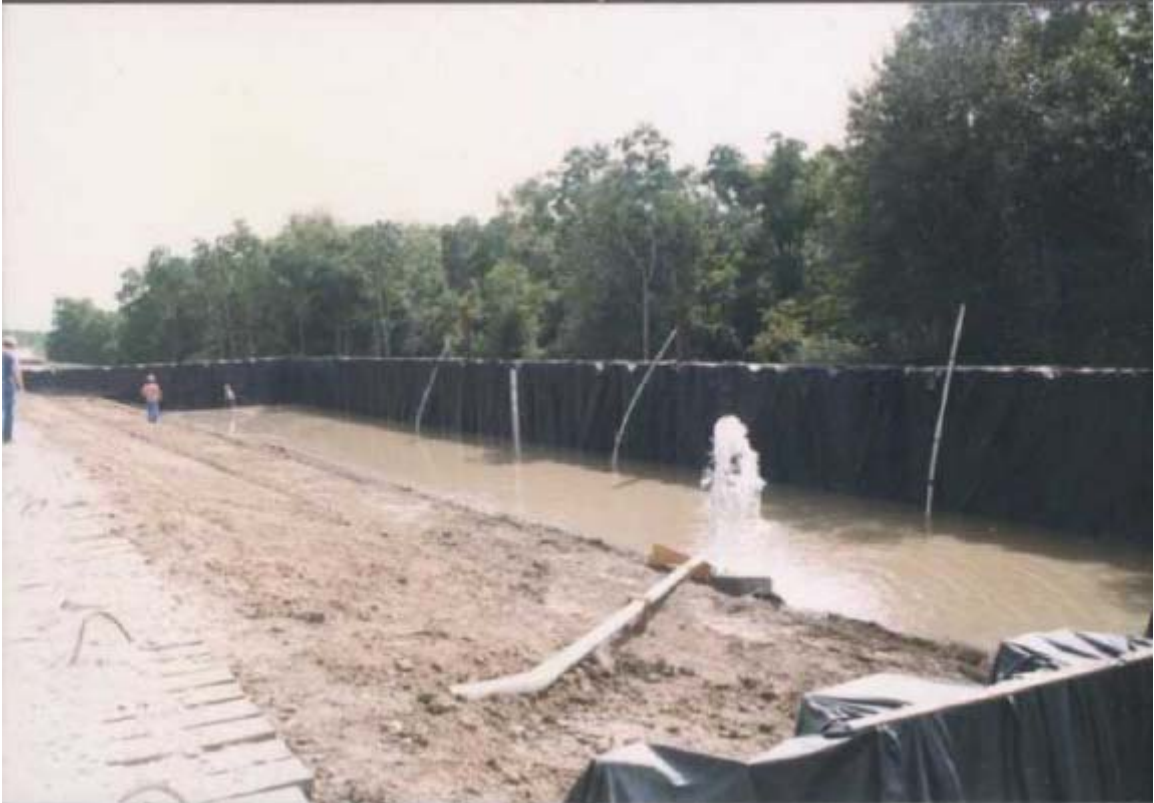
Figure 4-2: E-99 East Atchafalaya Basin Protection Levee Sheet Pile Wall Test
