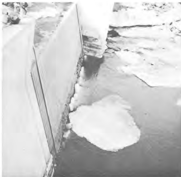
Floating ice against the trashracks. Note how the ice slabs have turned and flattened against the rack, greatly reducing the intake cross section. February 4, 1970. Photo CN66-436-828NA
