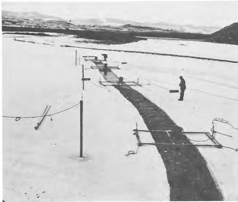
View looking upstream at channel cut in ice at the Wind River Diversion Dam. Four outboard motors and propellers have been placed in the channel to divert slush ice over the dam, thus preventing entry of ice into power canal. December 14, 1967. Photo P36-703-23NA
