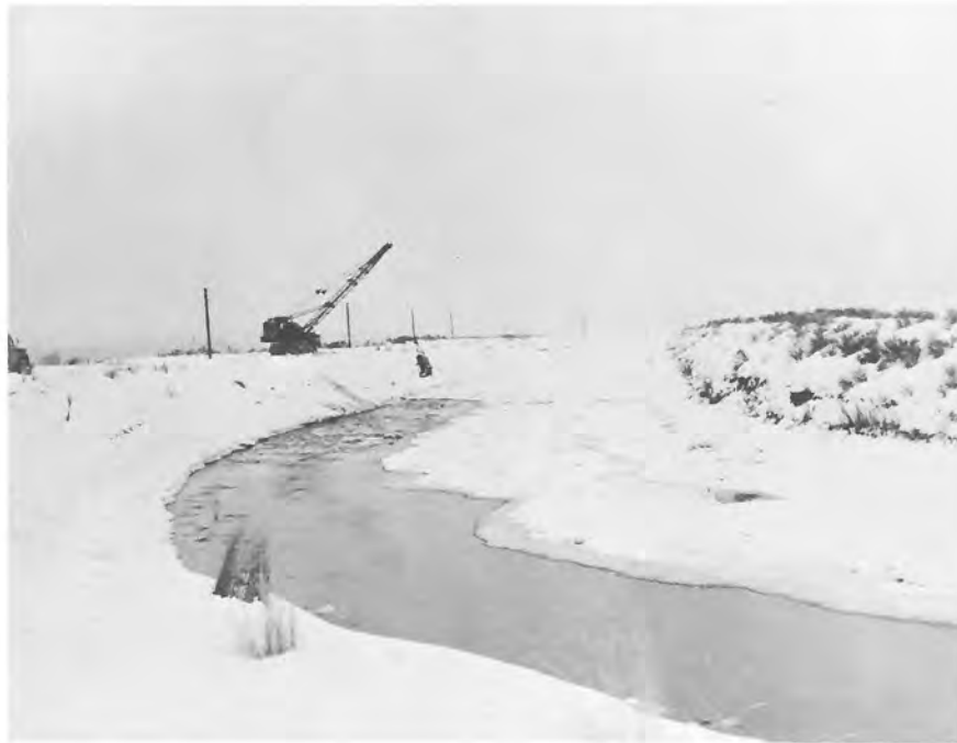
Roza I. D. breaking ice in Roza Canal at Mile 8, preparatory to starting Roza powerplant generator. Dragline can reach only half width of canal. January 11, 1965. Photo P33-109-6966NA
