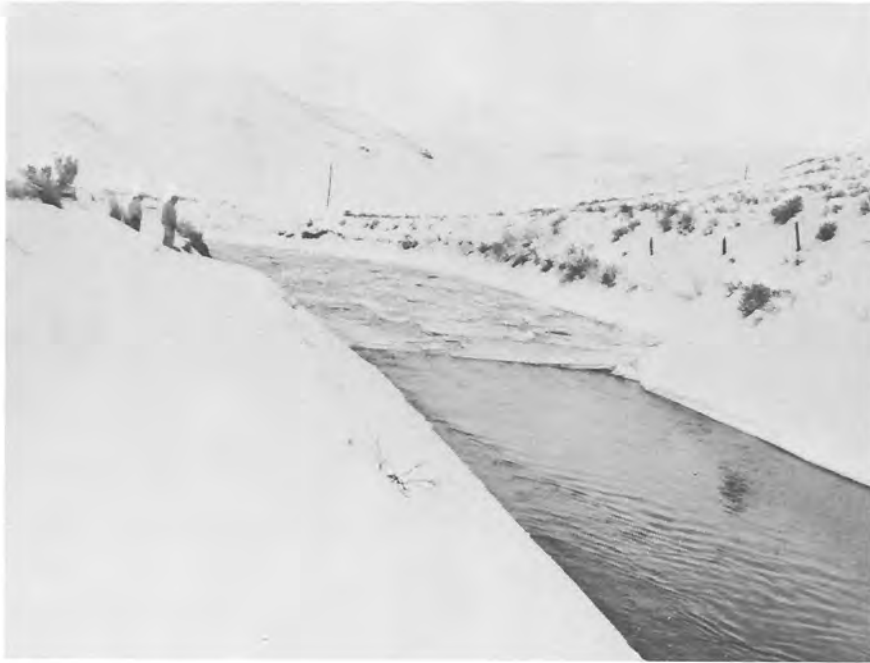
Lower end of ice jam in Roza Canal Mile 8.3, unlined to lined canal transition; flow 300 + cfs. January 7, 1965. Photo P33-109-6960NA
