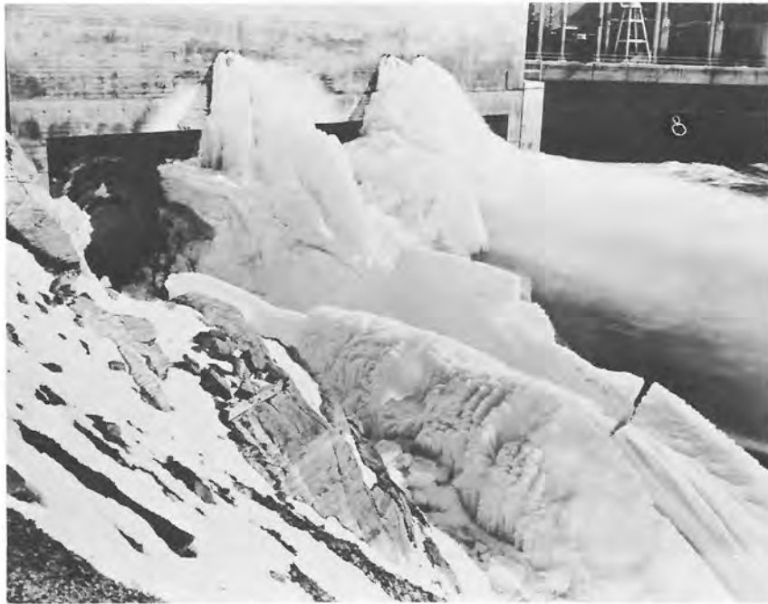
Closeup view of Hungry Horse outlet works showing ice buildup resulting from operation of the three 96-inch hollow-jet valves - No. 3 jet valve is still operating. March 23, 1965. Photo P447-105-6750NA
