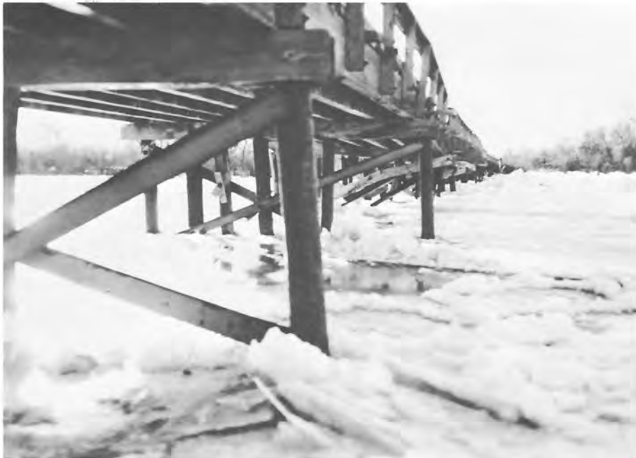
View showing stringers of Ervine Bridge on North Platte River, some broken by the ice. Upstream side of bridge. January 4, 1967. Photo P20-703-5715NA
