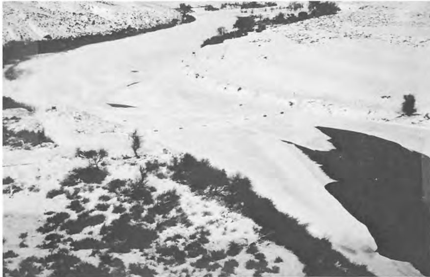
Log boom - North Platte River - North Platte Project - Wyoming. Panoramic view of log boom. January 4, 1971. Photo C20-703-1207
