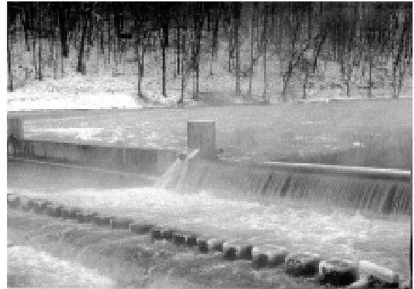
Figure 12. Ice control weir on Oil Creek, upstream of Oil City, Pennsylvania.
