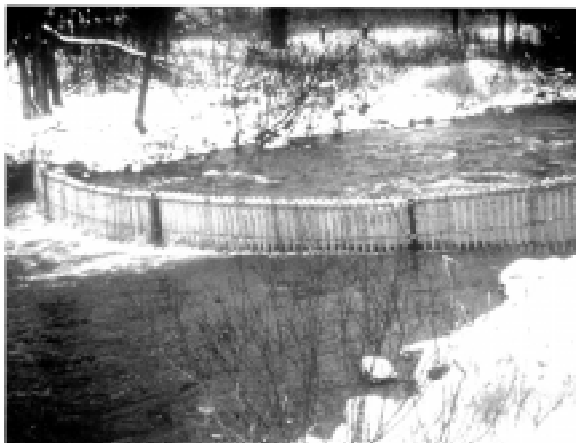
a. Installed condition.
