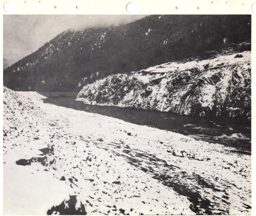
Photo 25. 29 October 1959. Completed spillway entrance looking upstream from about Station 30+00. Note high water line on trees about 50 feet above Earthquake Lake.
