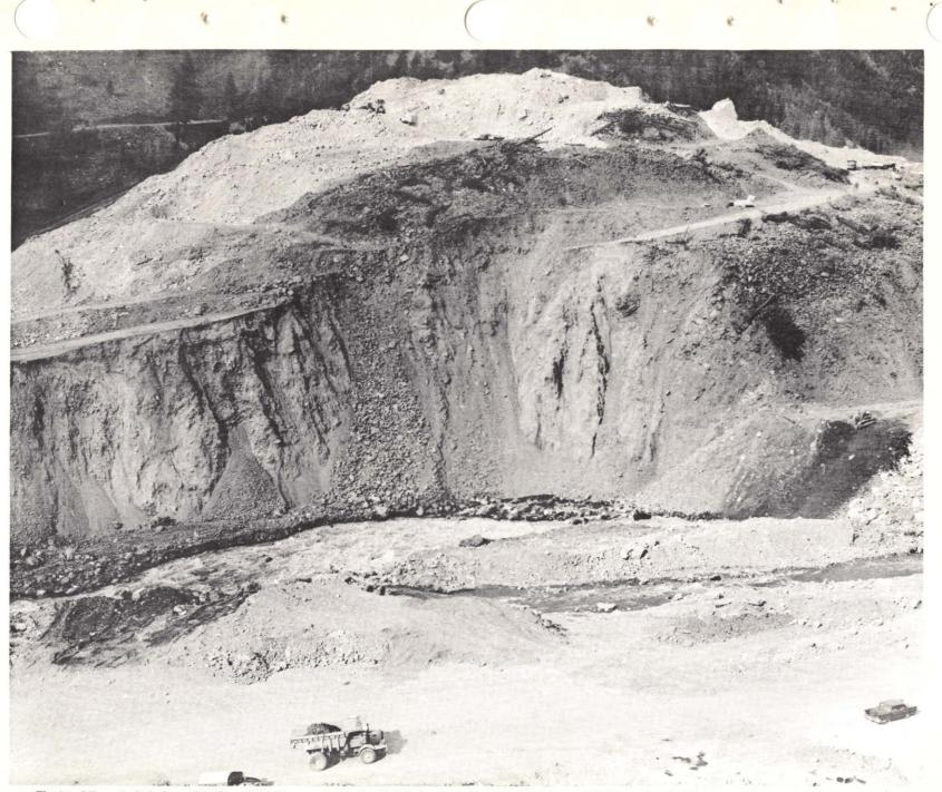
Photo 17. 5 October 1959. Rapid erosion of right bank between Stations 11+00 and 15+00.
