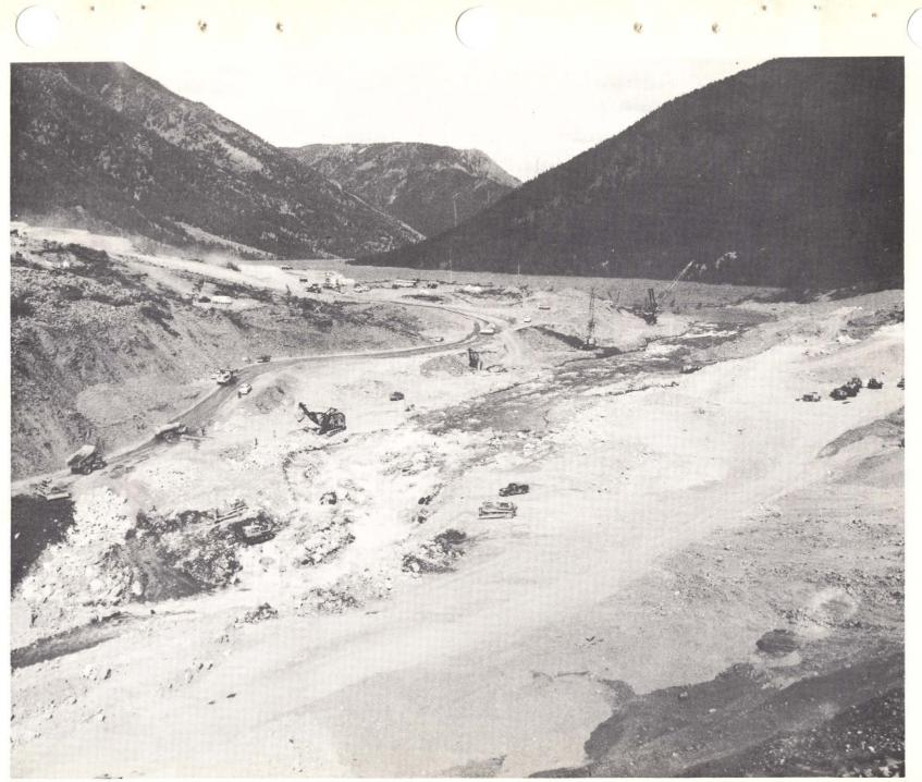
Photo 16. 5 October 1959. General view of spillway lowering operation. Draglines are working in channel and shovels are maintaining a work berm.
