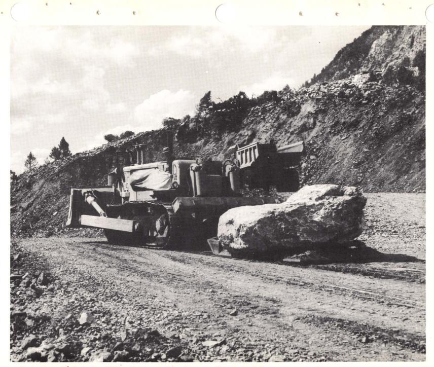
Photo 11. 16 September 1959. Tractor pulling large rock on rock sled.
