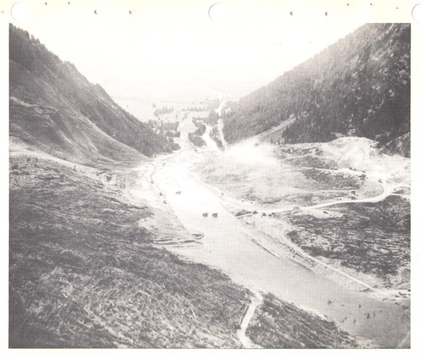
Photo 9. 11 September 1959. Downstream aerial view of water passing over slide in spillway channel.
