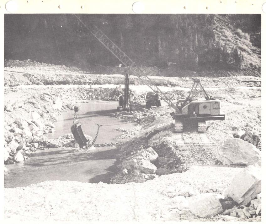
Photo 13. 16 September 1959. Foundation excavation for first rock filled drop structure at about Station 6+00.
