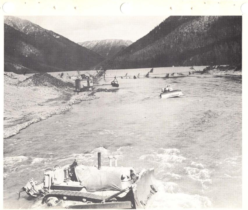
Photo 15. 29 September 1959. Starting to lower the spillway channel near the outlet of Earthquake Lake.
