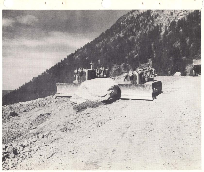
Photo 10. 11 September 1959. Two bulldozers pushing large rock.
