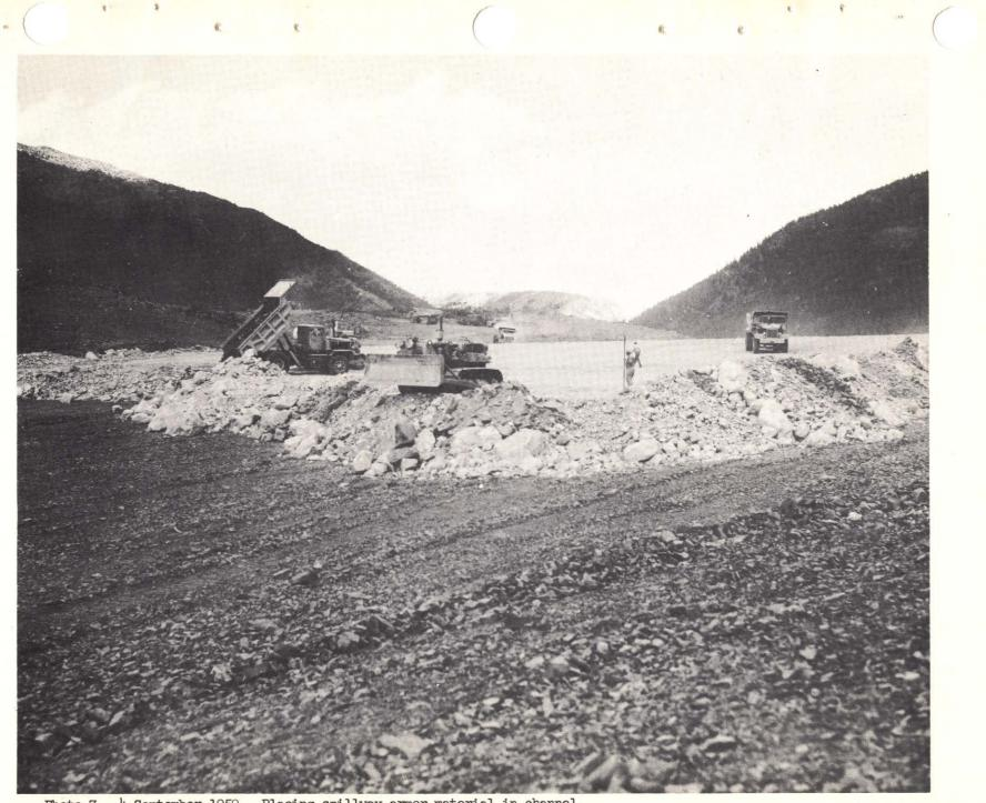
Photo 7. 4 September 1959. Placing spillway armor material in channel.
