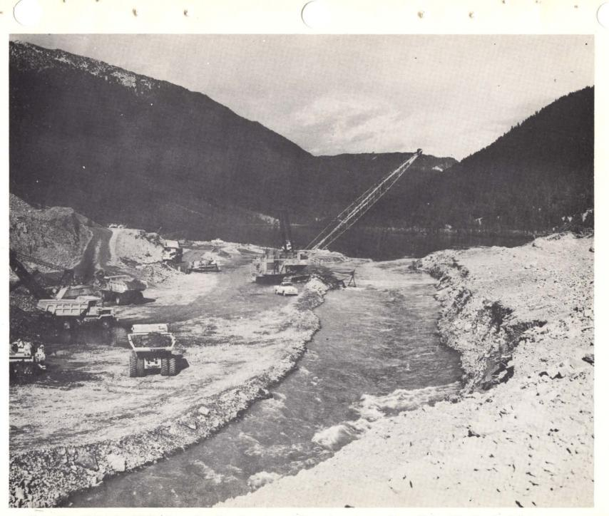
Photo 21. 11 October 1959. Large dragline lowering spillway channel near the outlet of Earthquake Lake.
