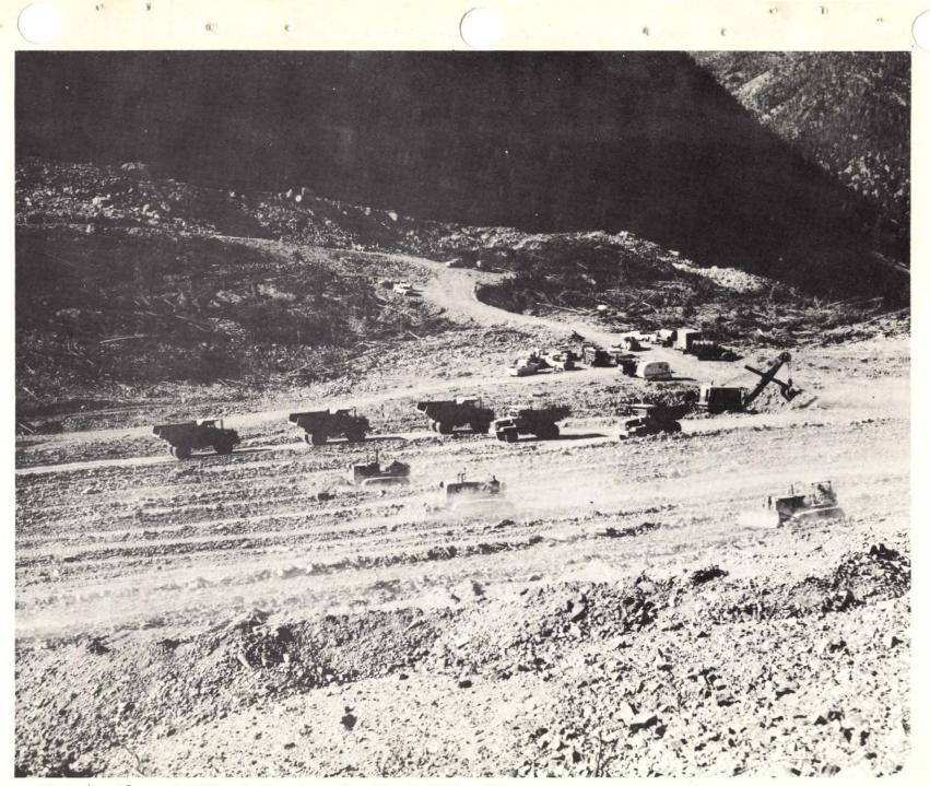
Photo 4. 28 August 1959. Equipment constructing initial spillway.
