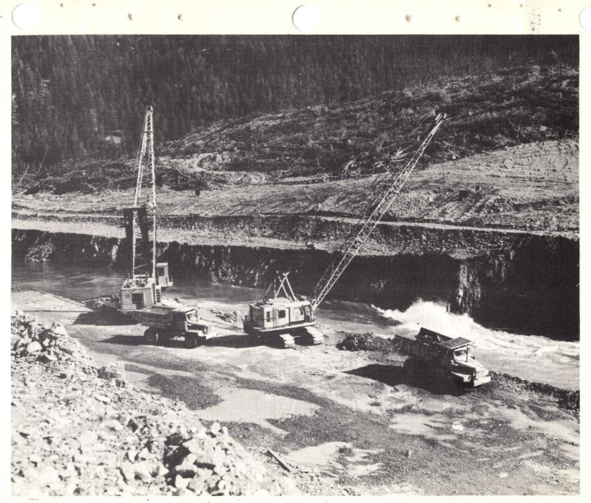
Photo 22. 14 October 1959. Draglines lowering spillway channel near Station 31+00.
