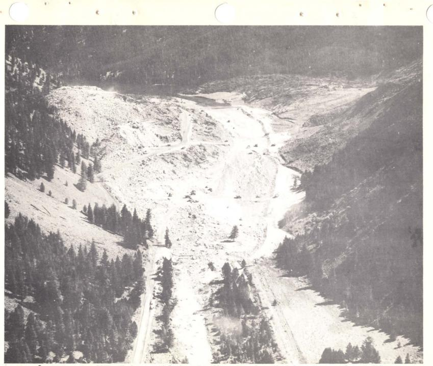
Photo 8. 10 September 1959. Upstream aerial view of spillway channel on first day water passed over slide.
