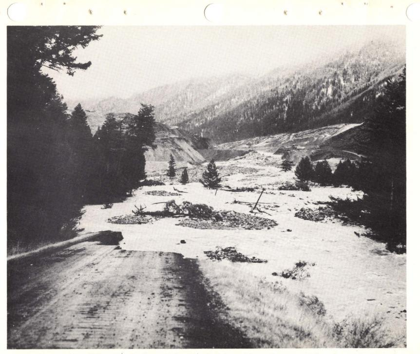
Photo 19. 9 October 1959. View showing rapid development of fan and damage to access road.
