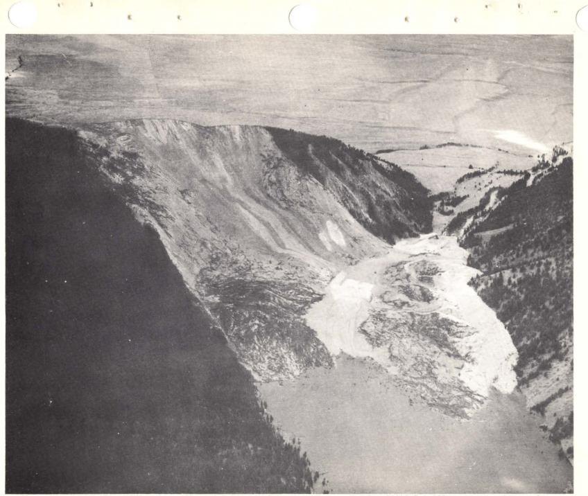
Photo 6. 3 September 1959. Over-all aerial view looking downstream showing initial spillway construction and a view of the slide scar.
