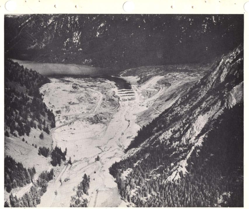
Photo 14. 22 September 1959. Aerial view of slide showing water pouring over rock terraces.
