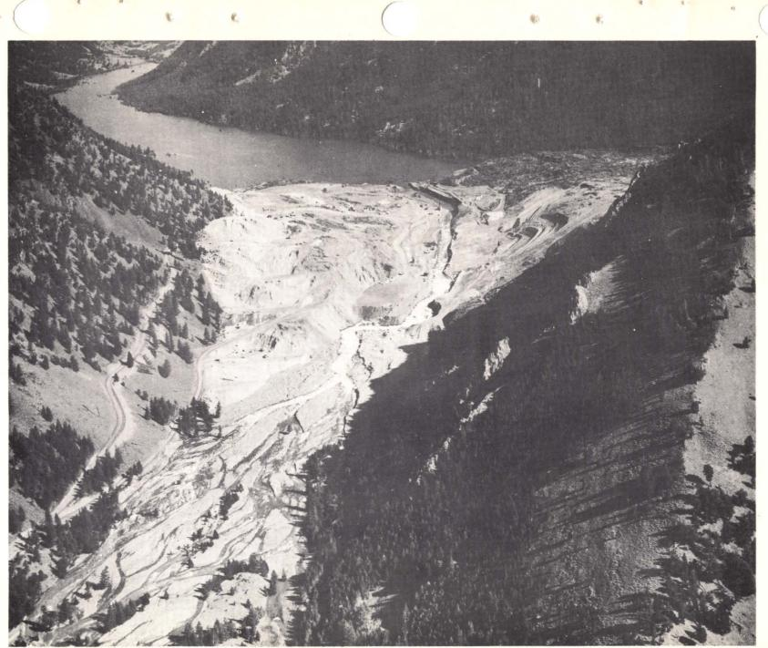
Photo 24. 17 October 1959. Aerial view of slide looking downstream showing spillway channel and buildup of fan below the slide.
