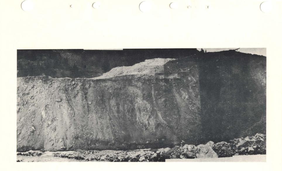
Panoramic view of right bank of slide spillway channel walls from approximately station 16 and downstream. Excessive lateral erosion occurred on right bank when water bypassed rock terraces in channel. Typical of material encountered in downstream reach of s illway. Photo taken 13 October 1959. (Photo #11)
