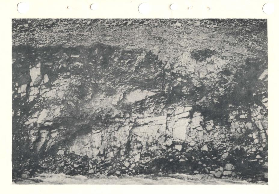
View looking at station 30 on left bank of slide spillway showing typical rock formations encountered in the upstream area during early stages of spillway lowering operations. Photo taken 13 October 1959. See photo #6 taken 23 October 1959 at same location, which shows massive rock formation becoming less apparent as lateral erosion progressed. (Photo #5)
