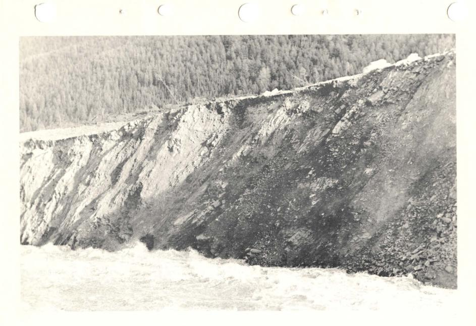
Oblique view of slide spillway taken from station 28 right bank at waters edge looking upstream with station 32 marker showing in picture. Picture shows rock and soil conditions of left bank. Rock formation shows through the light covering of dirt in the foreground. Water surface at station 30 approximately 6397 at time of picture. Photo taken 23 October 1959. (Photo #7)
