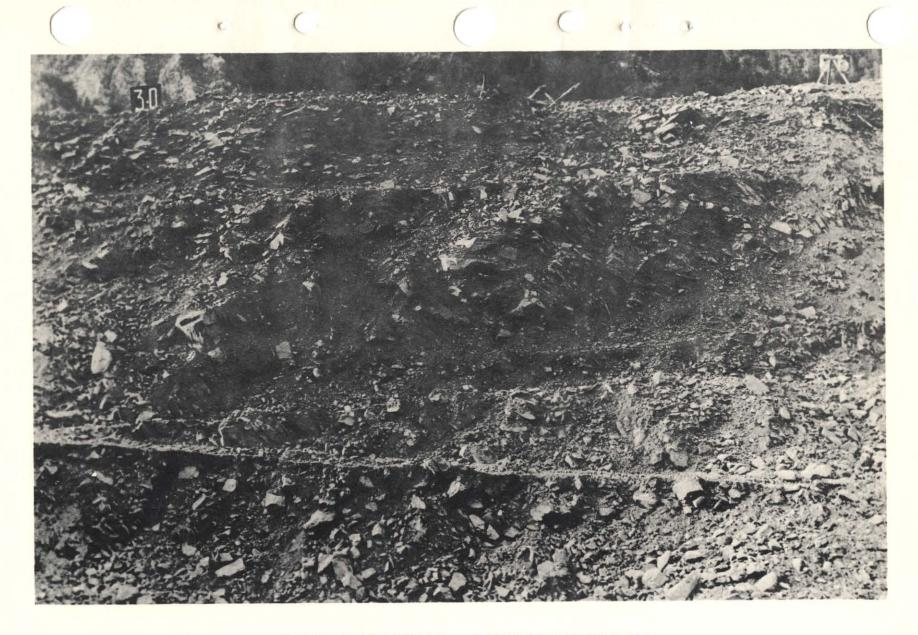
Oblique view of slide spillway taken from station 31 right bank at waters edge looking downstream at station 30 marker showing rock and soil conditions of right bank. Right bank was shovel excavated and most of rock formation covered with layer of loose rock and dirt. Note rock formation visible in several locations. Photo taken 23 October 1959. (Photo #10)
