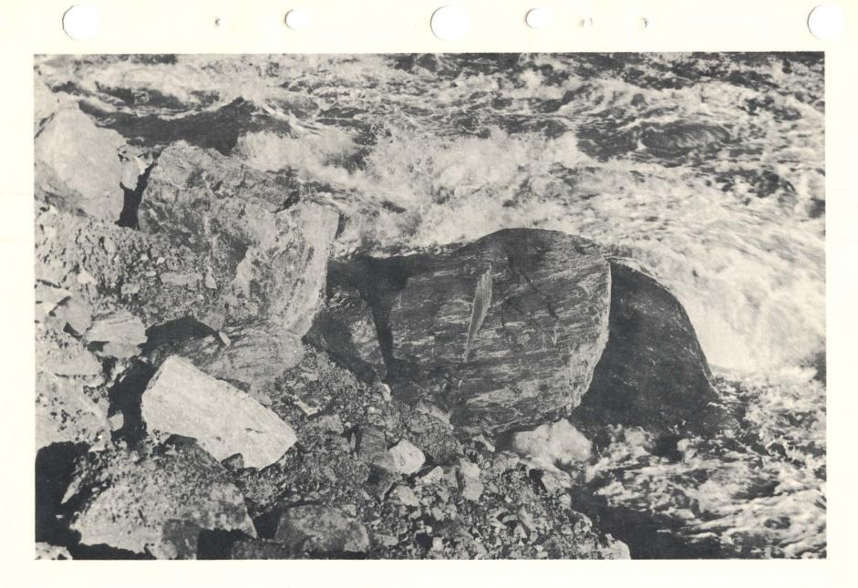
View showing the large gneiss rock which were dragged out of channel at station 26 to 26+50. Channel constricted at this location. Photo taken 23 October 1959. (Photo #8)
