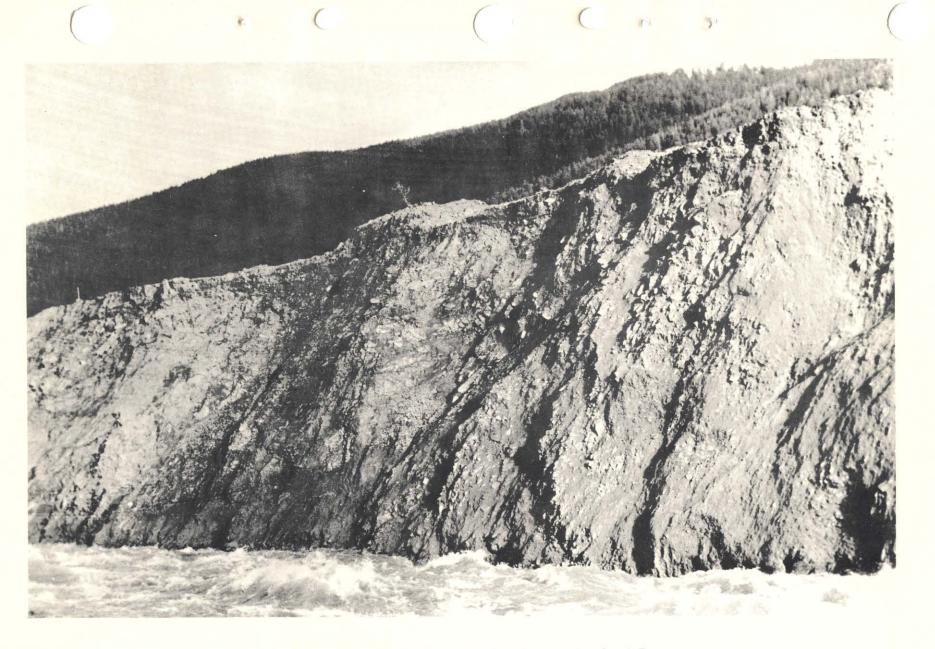
Oblique view of slide spillway taken from station 30 right bank at waters edge looking upstream showing rock and soil conditions of left bank. Lateral erosion was extensive at this location and rock formation became less apparent as erosion progressed. Photo taken 23 October 1959. (Photo #6)
