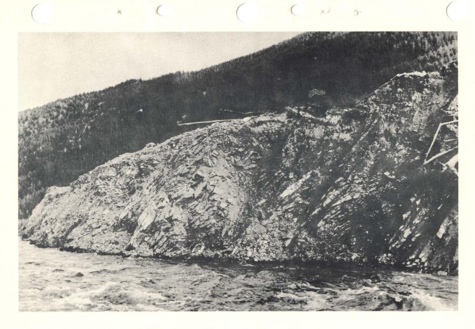
Oblique view of slide spillway taken from waters edge at station 35 looking upstream to lake entrance. View shows the rock and soil conditions of the left bank at this location before the start of bank sloughing from lateral erosion. Water surface of lake approximately 6412. Photo taken 23 October 1959. (Photo #2)
