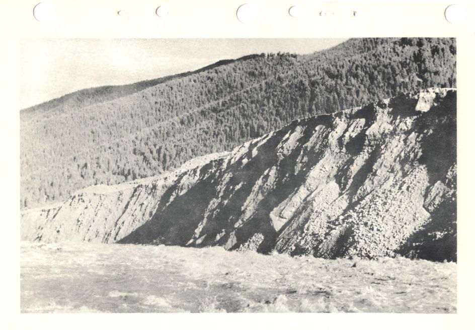
Oblique view of slide spillway taken from station 19 right bank looking upstream showing rock and soil conditions of left bank. Material "Earthy" with occasional boulders and very susceptible to erosion. Typical of downstream reach of spillway. Light bank at top the original 10 foot rock lining of spillway. Photo taken 23 October 1959. (Photo #12)
