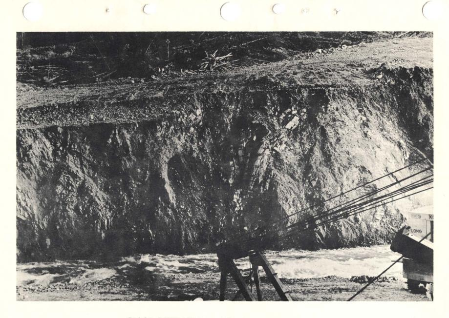
Oblique view of slide spillway taken from station 32 right bank looking upstream to station 34 left bank, showing the rock and soil conditions. Top earthy material tended to cover the rock formation as lateral erosion progressed. Water surface at station 34 approximately 6404. Photo taken 23 October 1959. (Photo #4)
