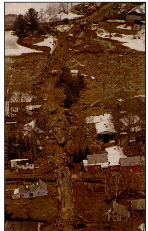
Fig. 6 – Route 140 after the Flood
