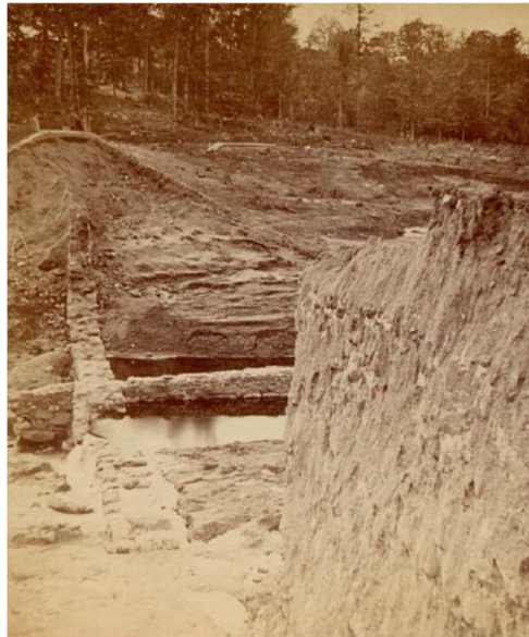
Figure 48: Remnants of the Mill River Dam in Williamsburg, MA after its breach, 1874. Source: Wooten et al. (2014).
