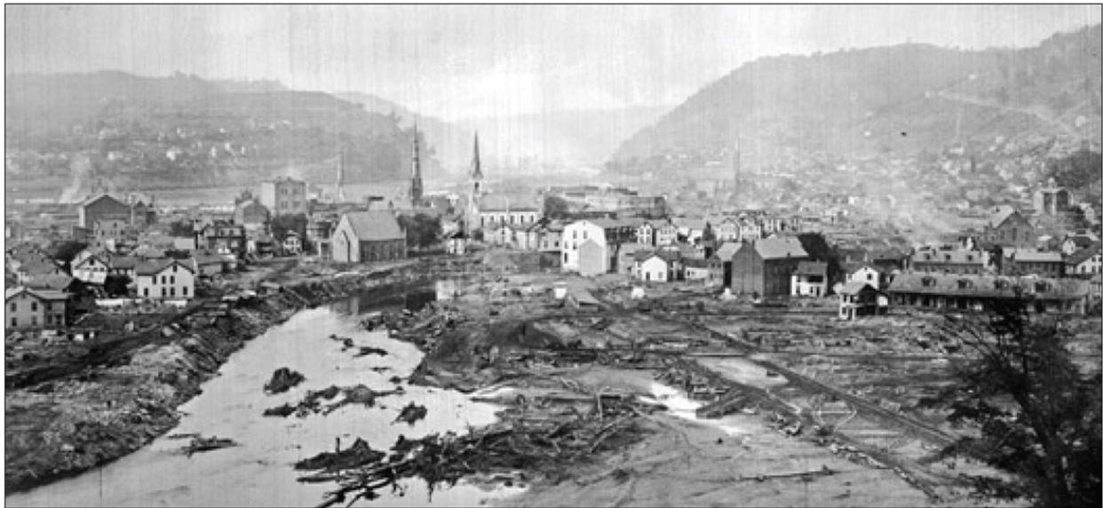
Figure 41: Johnstown after months of post-flood clean-up, 1889. Source: Hanna (2021).
