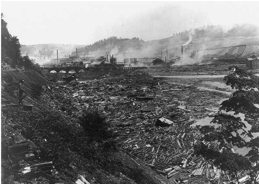
Figure 38: Debris jam at the Stone Bridge after the fire. Source: Lindberg (2024).
