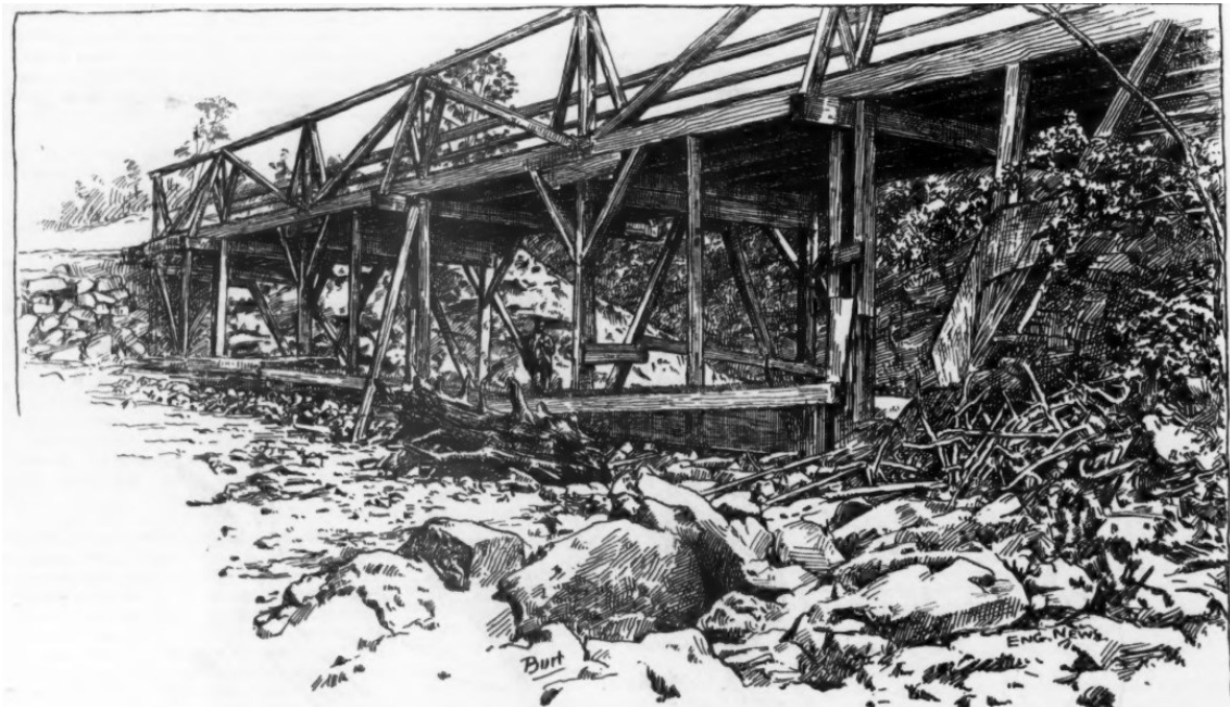
Figure 27: Contemporary illustration of the debris-laden fish screen remnants at Lake Conemaugh's spillway after the South Fork Dam breach. Source: Wellington and Burt (1889 B).
