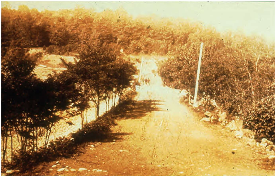
Figure 22: The South Fork Dam's crest looking southwest, 1880s, with its perceptible central sag. Source: Hanna (2021).
