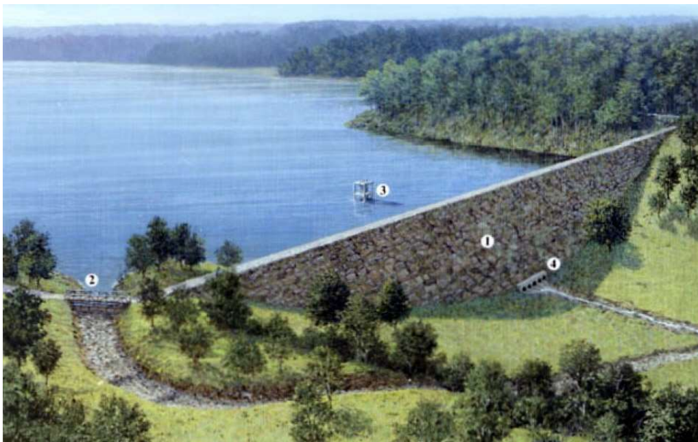
Figure 8: The Western Reservoir dam, 1853-1862. Note its (1) sturdy construction with downstream riprap, (2) northeast spillway, (3) control tower, and (4) discharge culvert. The drawing erroneously omits the southwest spillway and shows the culvert with five openings rather than one. Source: NPS (2023 C).
