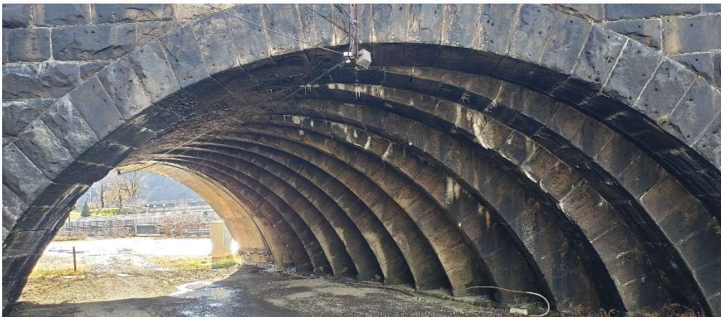
Figure 37: Close-up of one of the Stone Bridge's ribbed arches. Source: Author.
