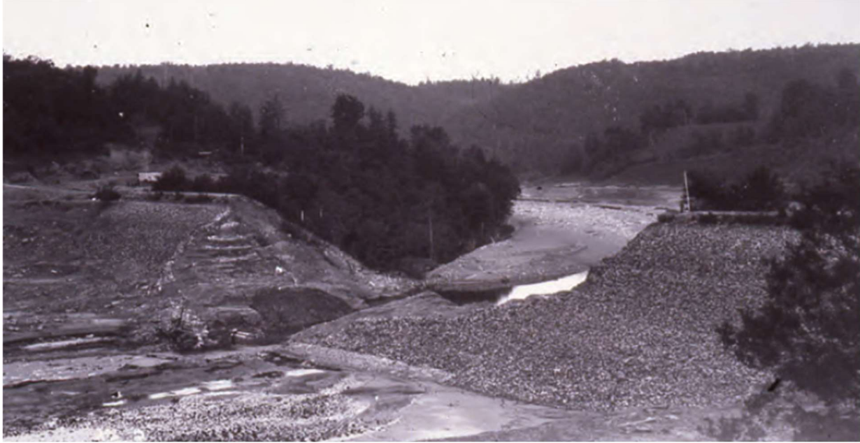
Figure 43: Former bed of Lake Conemaugh and remnants of the South Fork Dam looking downstream, 1889. Source: Hanna (2021).
