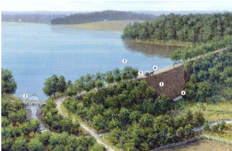
Figure 16: The South Fork Dam, 1881-1889. Note its (1,6) poorly rebuilt breach, (2) northeast spillway with fish screens and log boom, (3) lack of a control tower, (4) abandoned discharge culvert, and (5) lowered crest. Source: NPS (2023 C).
