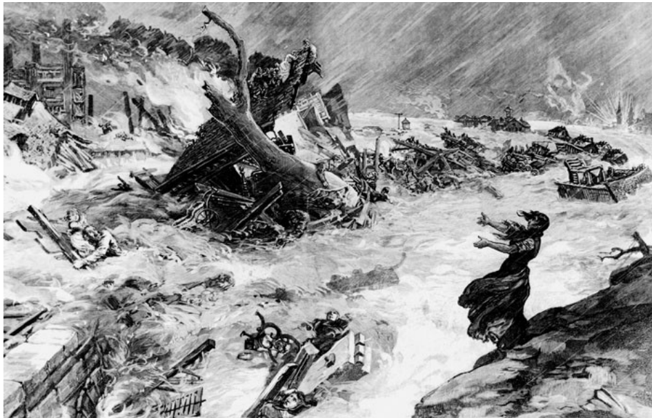
Figure 32: Contemporary lithograph of the 1889 flood on its deadly rampage. Source: JAHA (2024 B).
