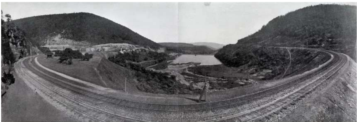
Figure 10: Panoramic view of the Horseshoe Curve near Altoona, PA, in the late 1800s. Its westbound (left to right) ascent is clearly visible. Source: Smolka (2022).
