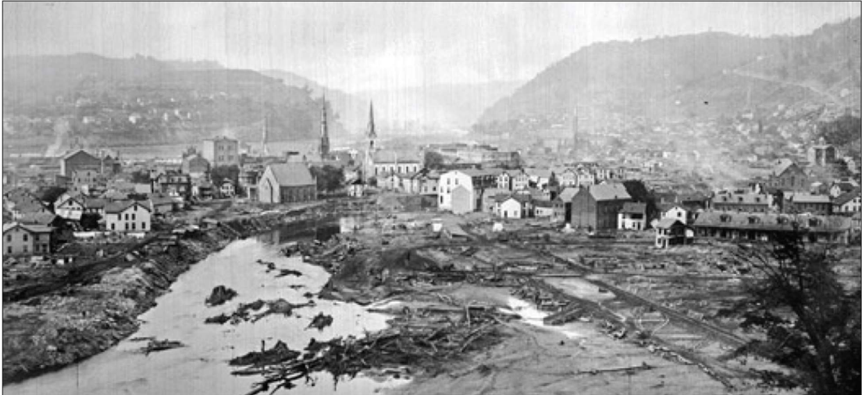
Figure 41: Johnstown during the early weeks of rebuilding, 1889. Source: Hanna (2021).
