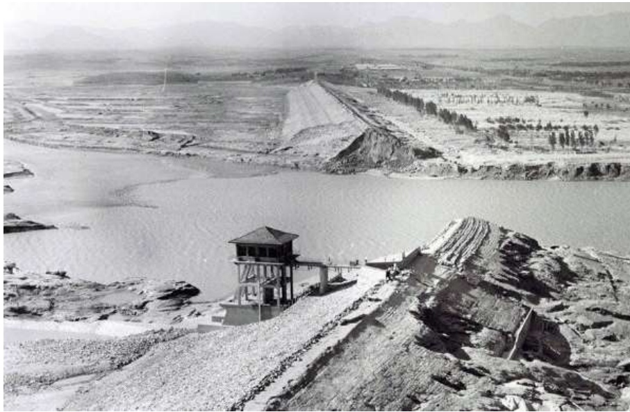
Figure 50: Remnants of the Banqiao Dam in China after its breach, 1975. Source: Lynch (2023).
